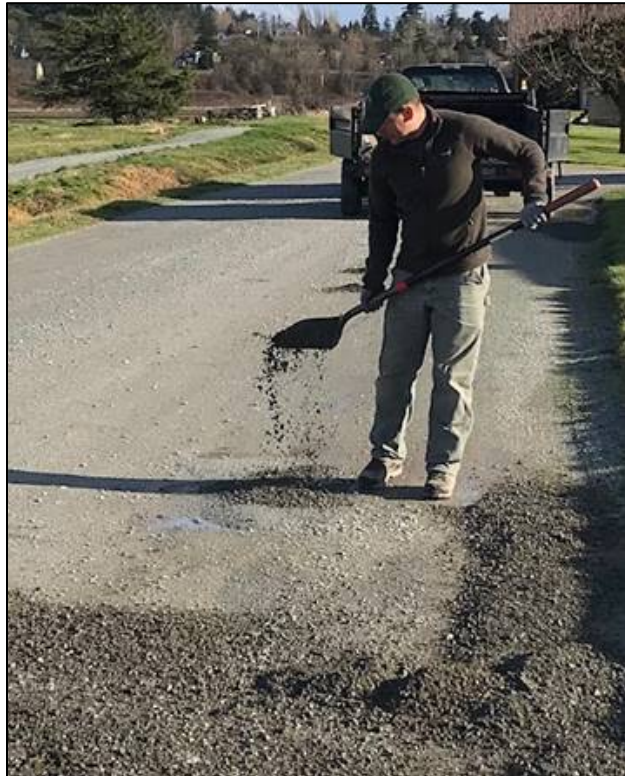
Repairing potholes at a Waterfowl Quality Hunt Program parking spot
