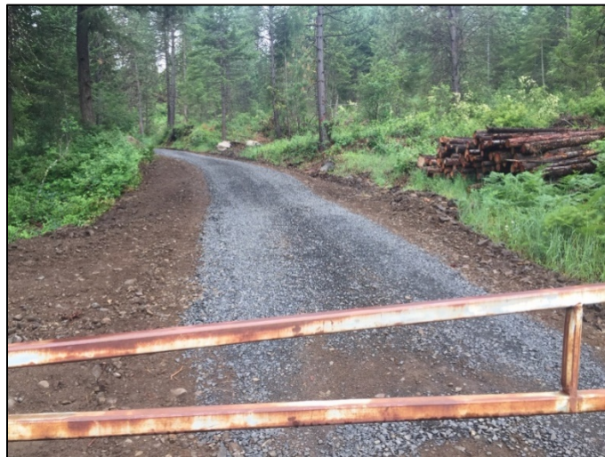
New gravel laid down by WDFW engineers
