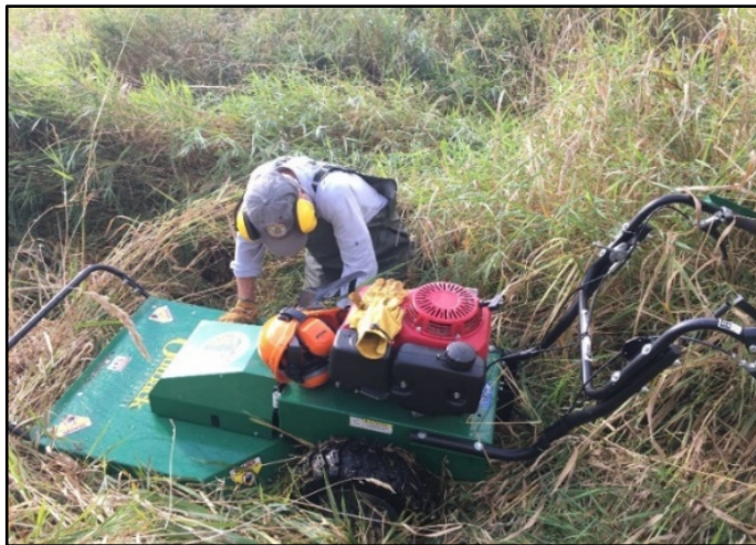
Testing the limits of the equipment
