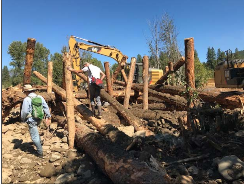
Large woody debris structure in the North Fork Teanaway River
