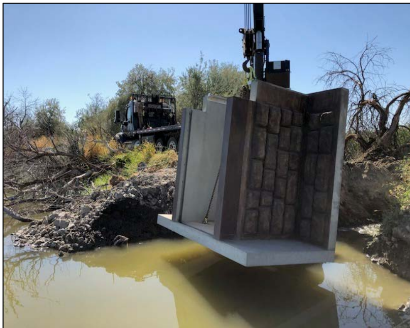
Water control structure almost in place
