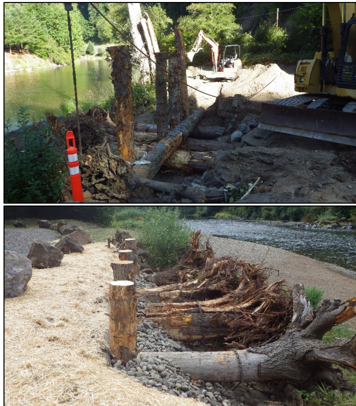
Bank stabilization at Beginners Hole Access
