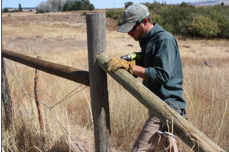
Finishing end brace by Cattleguard
