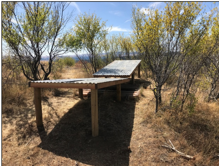
Guzzler C roof finished
