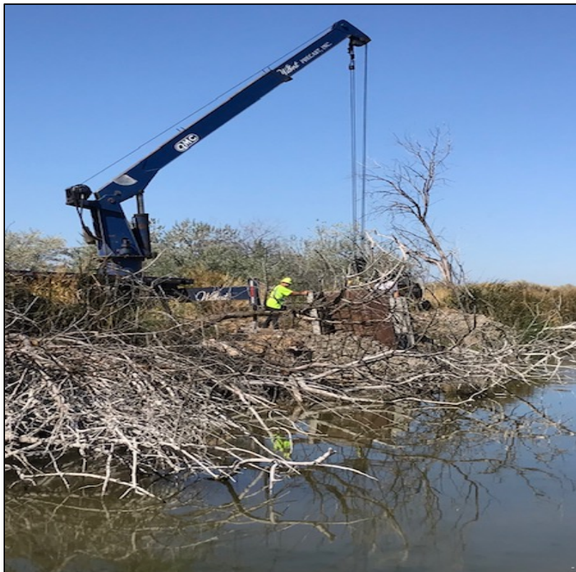
New water control structure being lowered into place at Windmill Lake
