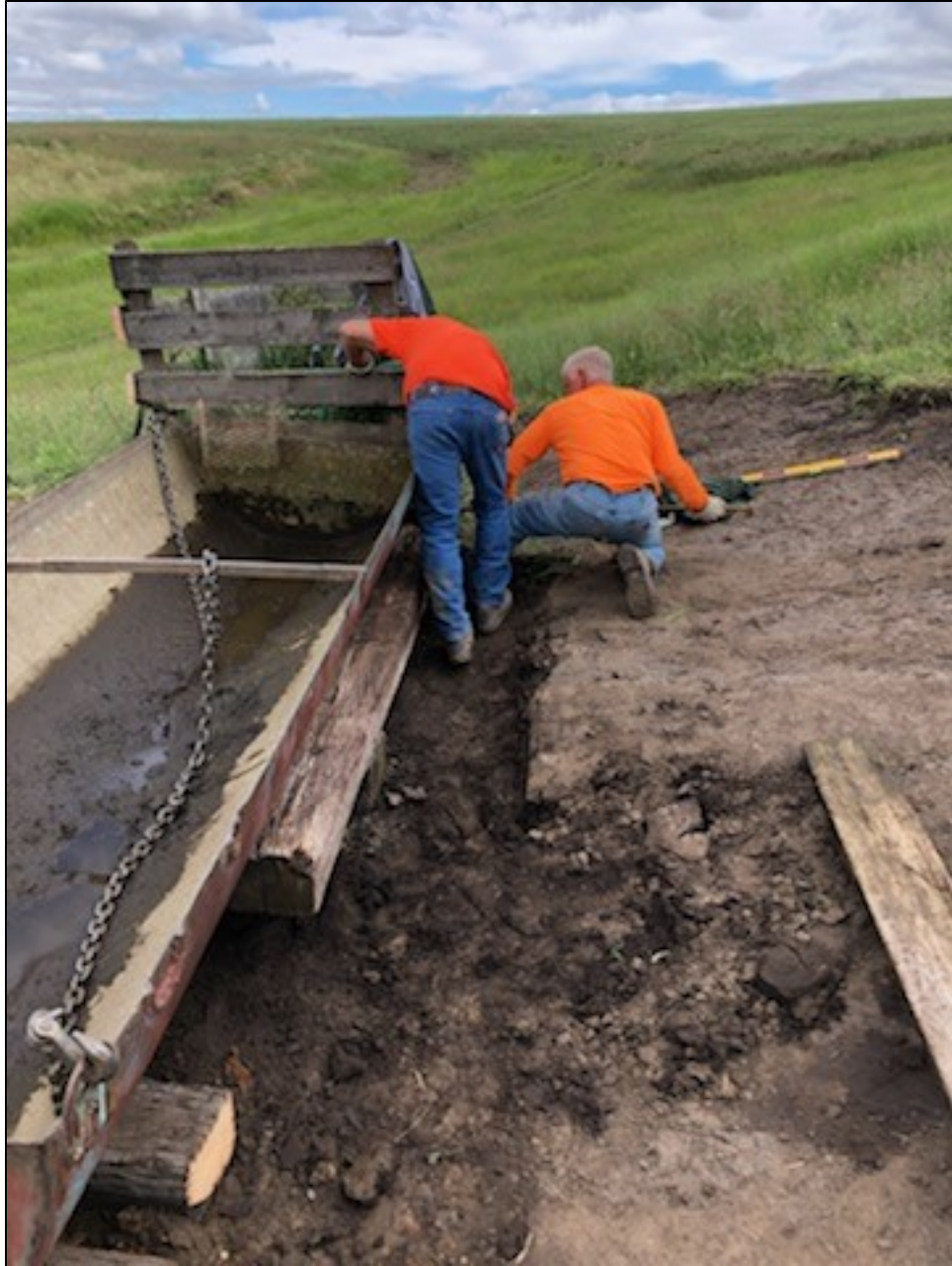
Technicians Dave Meisner and Scott McGee resetting a trough on railroad ties at Smoothing Iron Ridge where the trough is heavily used by elk
