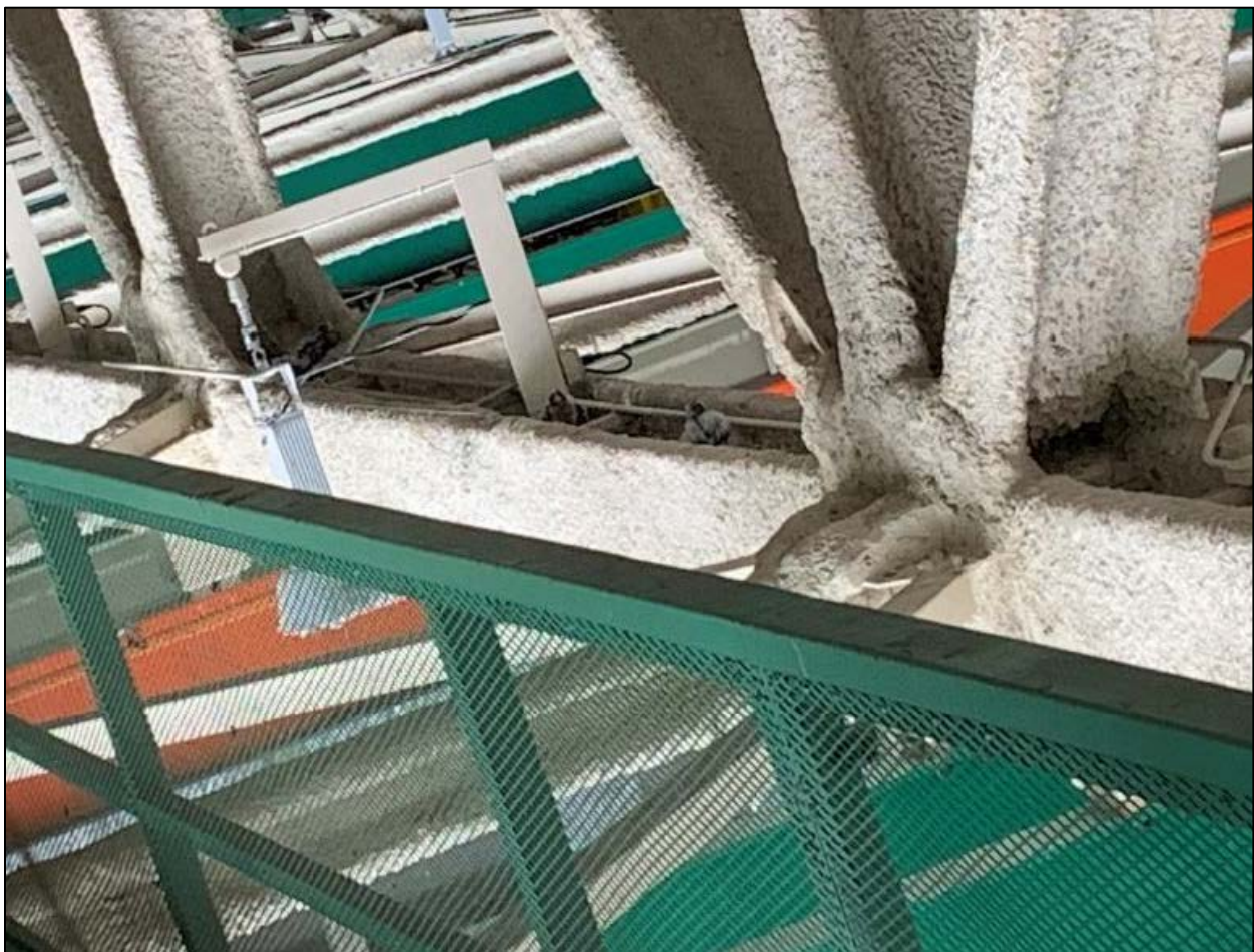
Falcon chicks being removed from their nest in the beam infrastructure inside a factory. Note helmets. Chicks were placed with falconers. This avoids safety issues both for humans within the factory but also for the fledging chicks who have broken wings and other injuries due to poor navigation of the factory environment in the past. Birds unharmed and get to hunt in the wild. - Photo by Boeing
