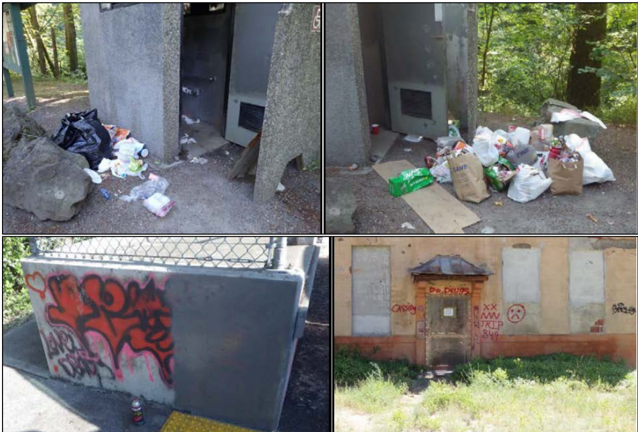
Trash and Graffiti at Barbers, Langsdorf, and Icehouse Access Sites
