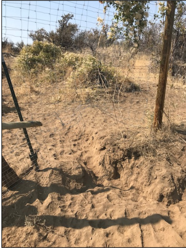
Damaged fence allowing elk to get into a crop field
