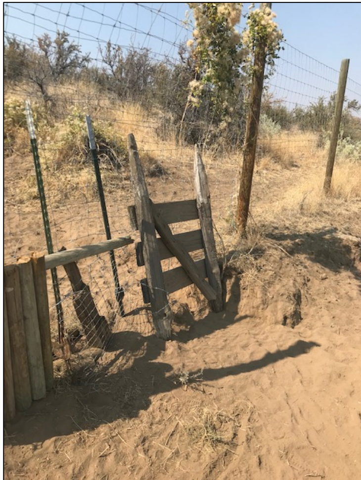
Temporarily repaired private elk fence
