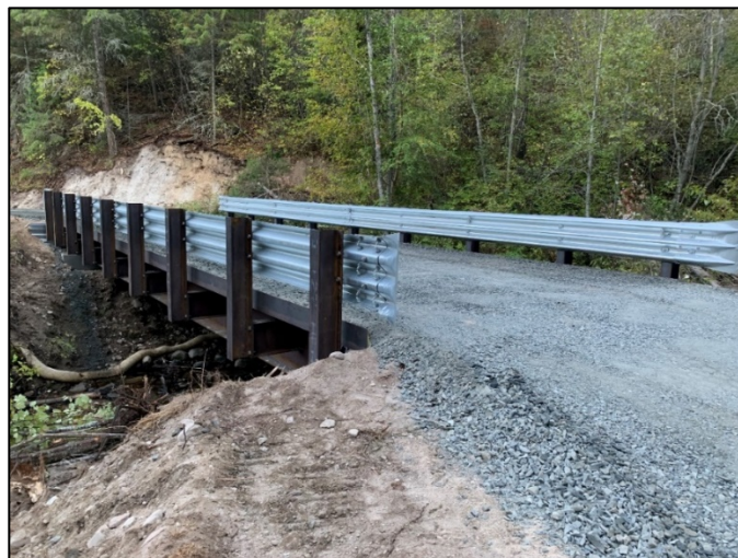
The bridge installed over Trout Creek in cooperation with BPA
