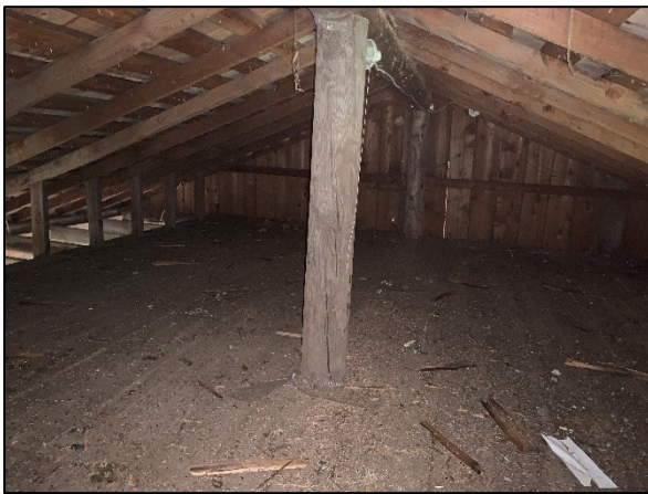
Attic space in the structure
