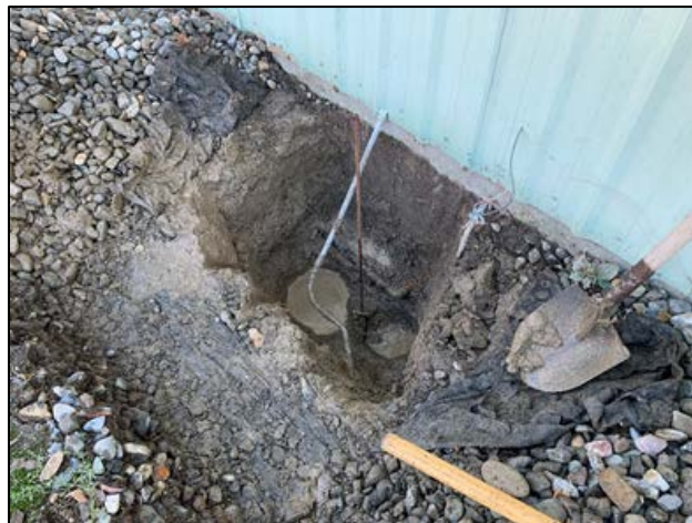
Hole dug for valve replacement
