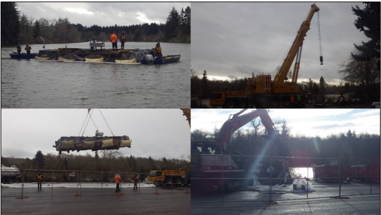
Removal and disposal of derelict barge at Oneida Access Site
