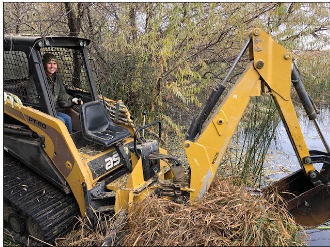
Assistant Manager Rodgers restoring water flow
