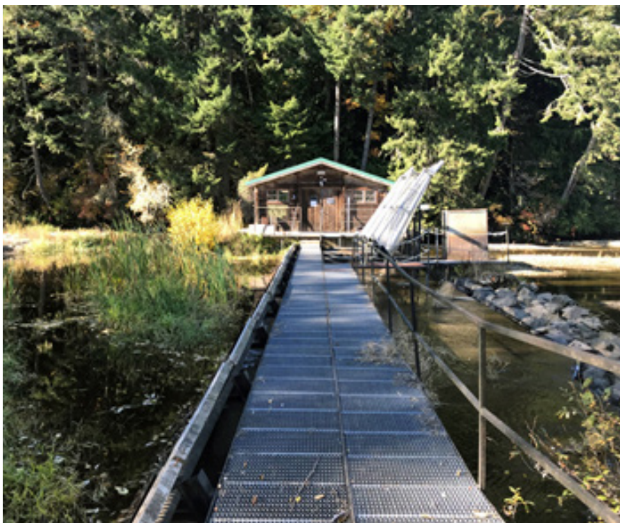
WDFW Fish weir – Big Beef Creek. Photo by Darric Lowery.
