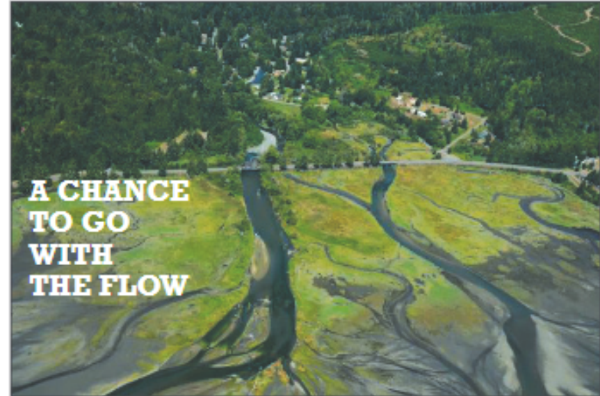
An aerial view of the Duckabush Estuary showing US Highway 101 and the two bridges that will be replaced. Photo courtesy of the Washington Department of Ecology.
