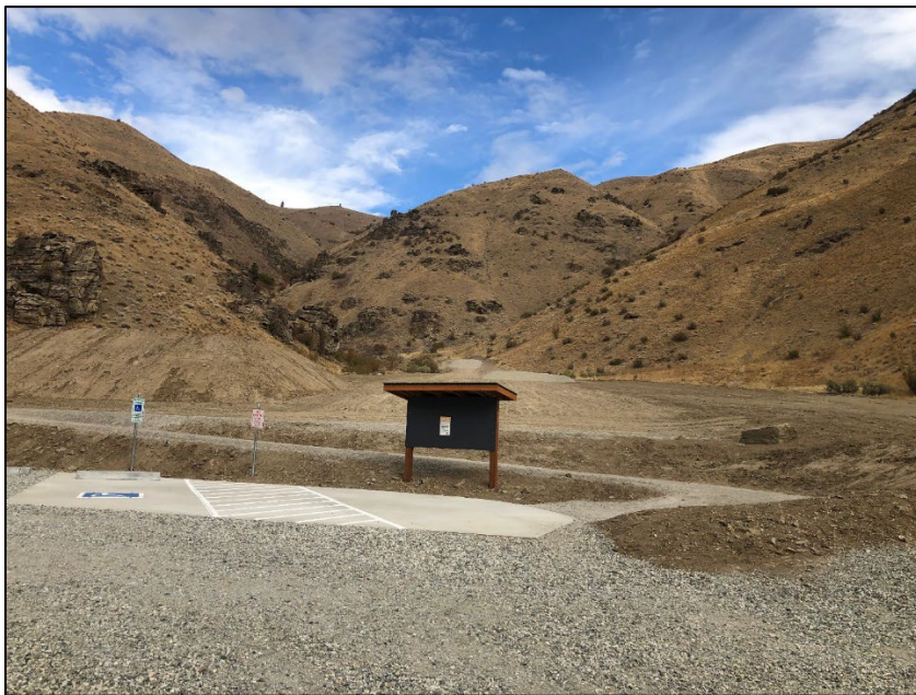
Swakane target shooting range at the completion of Phase 1.
