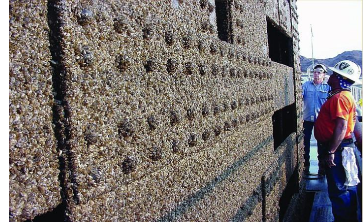
Invasive mussels fouling a penstock gate at Davis Dam. 📷: U.S. Bureau of Reclamation
