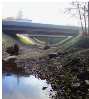
WSDOT completed $8.7M fish passage project in 2017.
