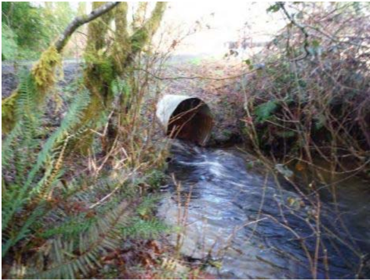
127Y0374 Before: 4ft by 25ft round culvert
