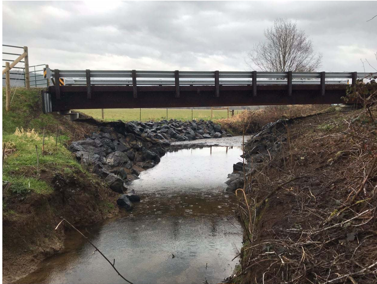
After: 60ft steel bridge
