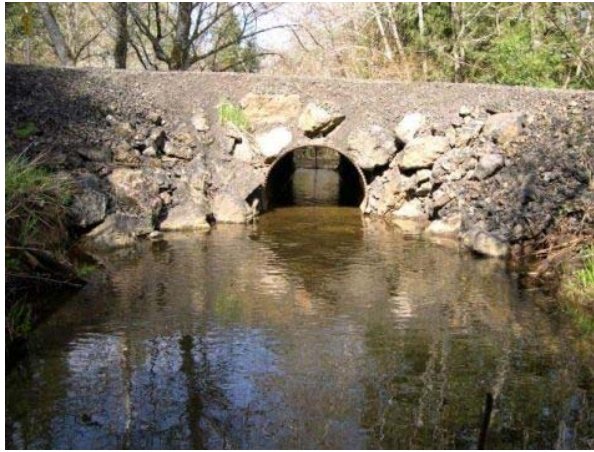
103-1022 Before: 4ft x 35ft round culvert
