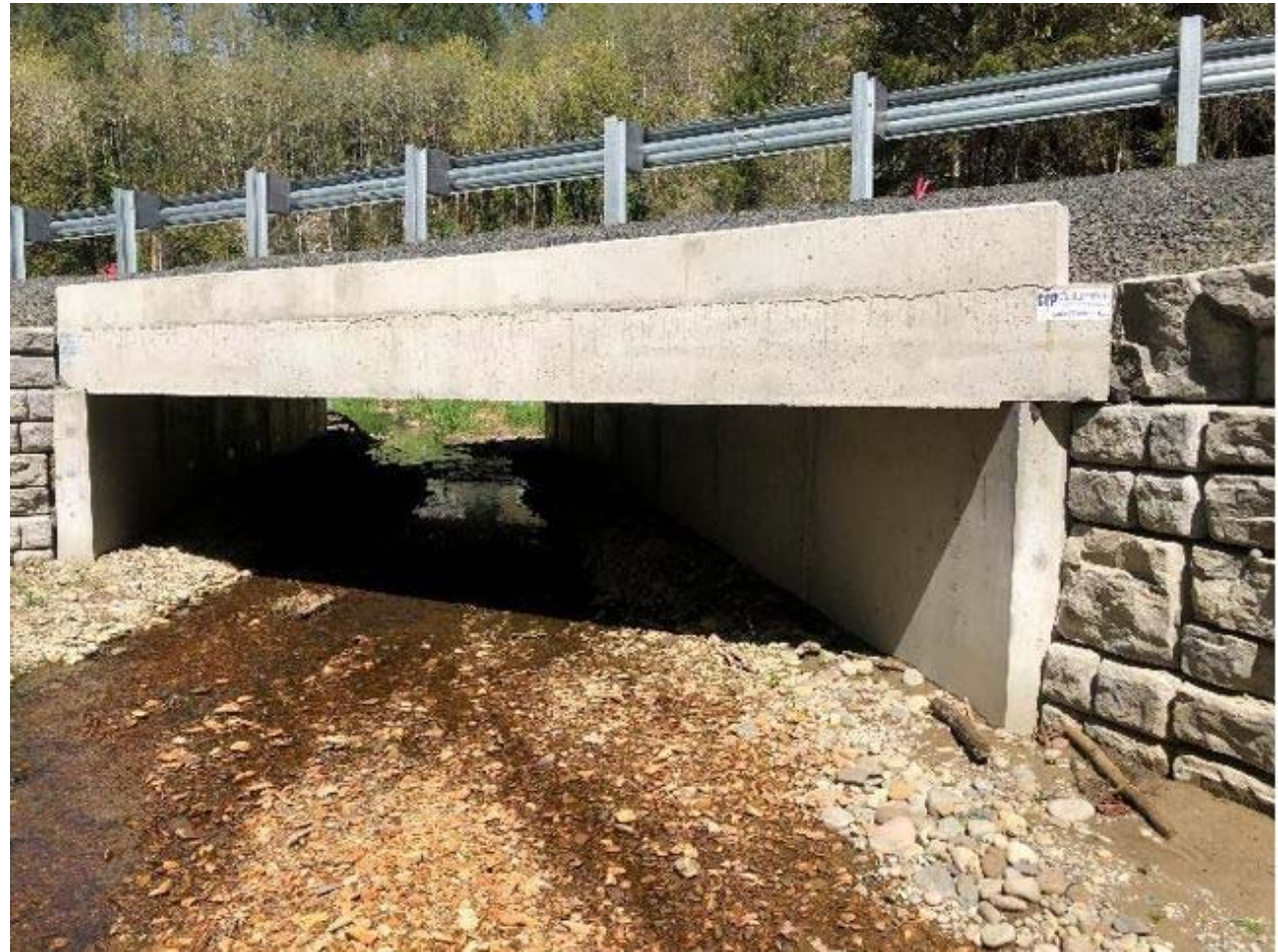
After: 16ft x 8ft x 36ft Box Culvert
