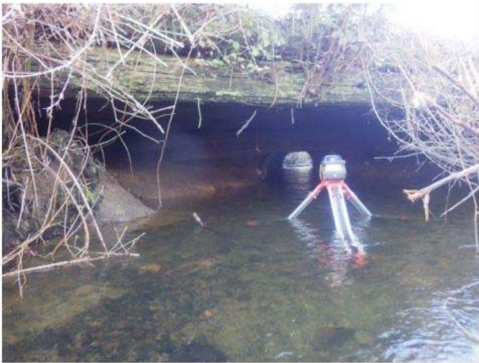
127Y0316 Before: 5ft x 40ft round culvert
