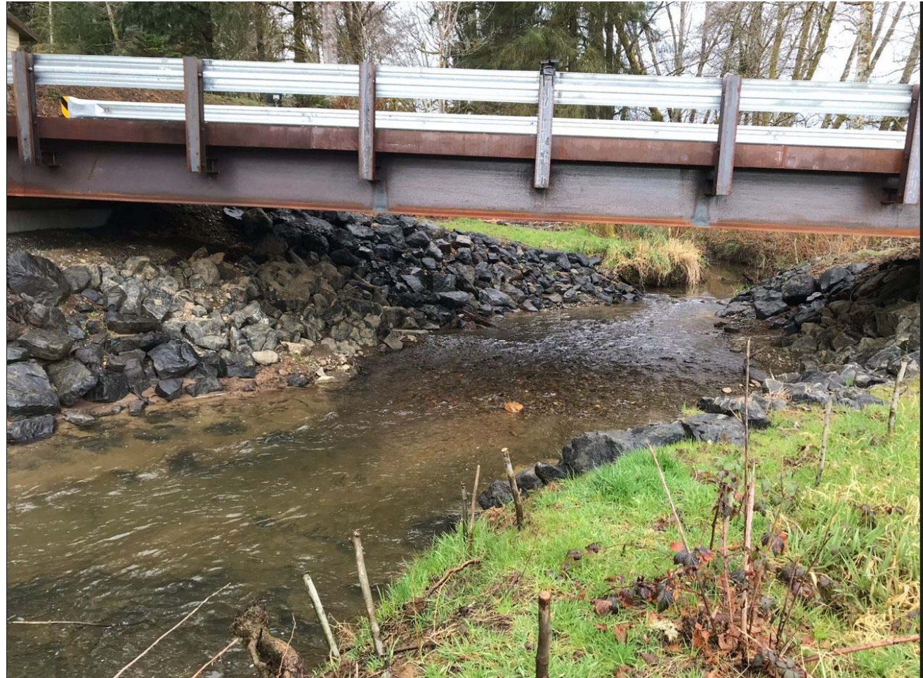
After: 50ft Steel Bridge
