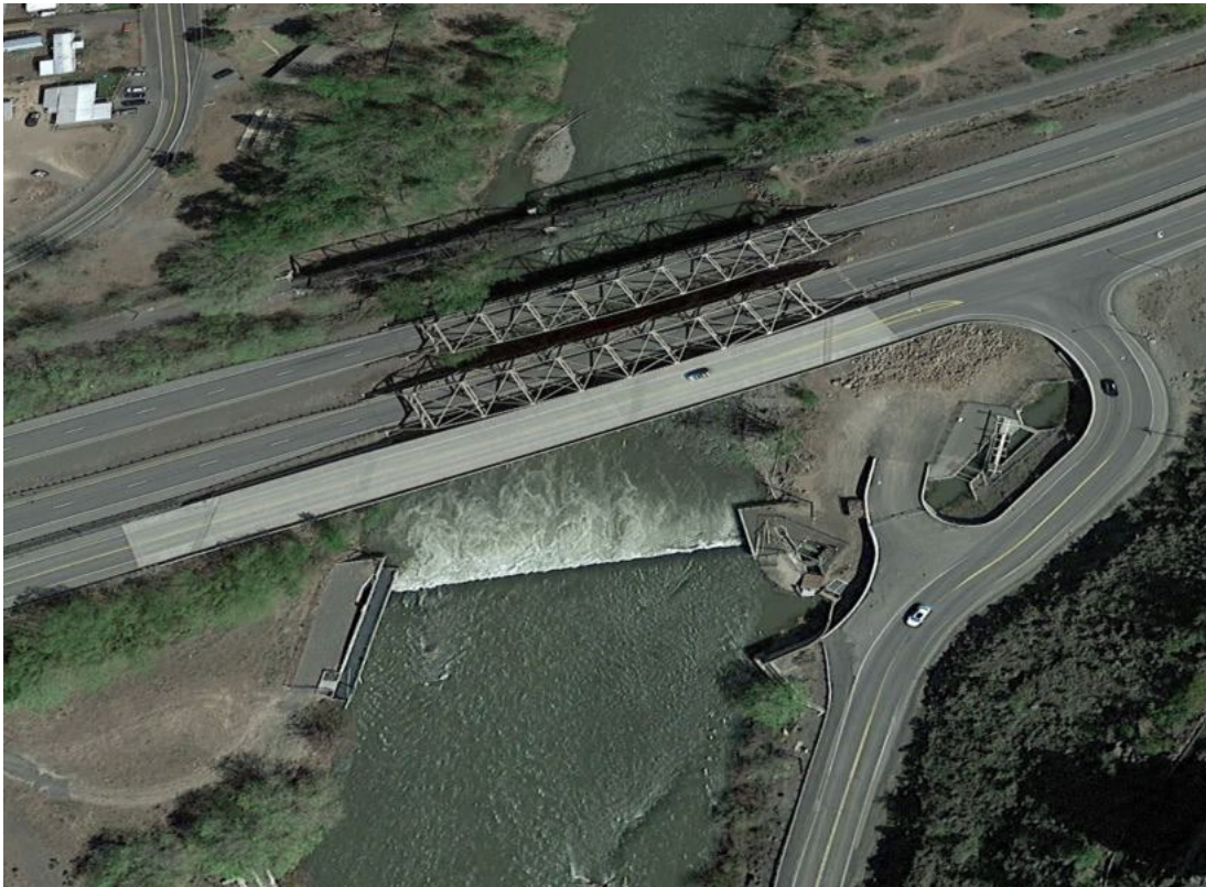
Before: 33% passable barrier, 180 ft. by 8ft., full span concrete dam.
