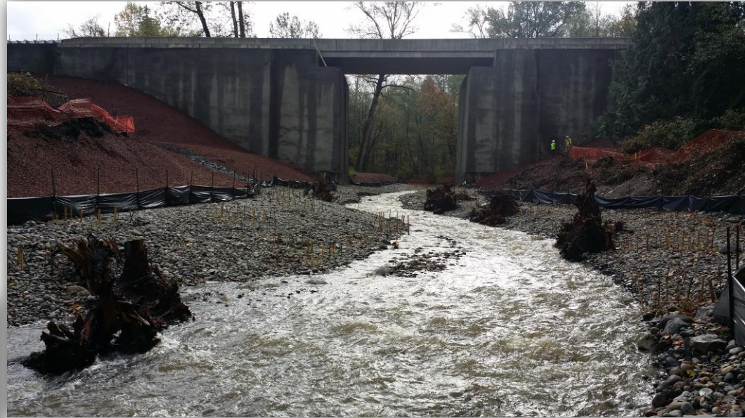
42 ft wide bridge
