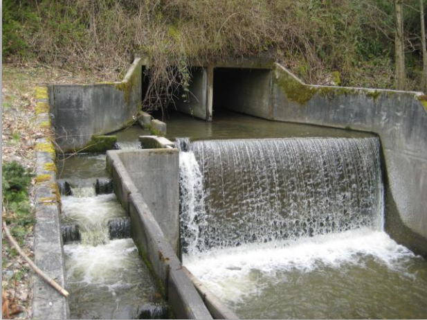
Two 8 ft box culverts and fishway
