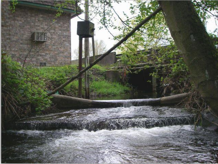
Twin 5 ft wide box culverts
