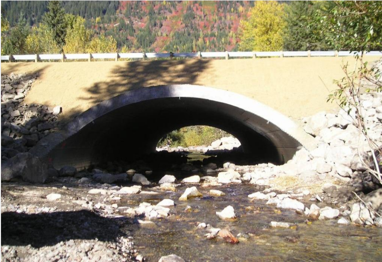
Stream simulation culvert
