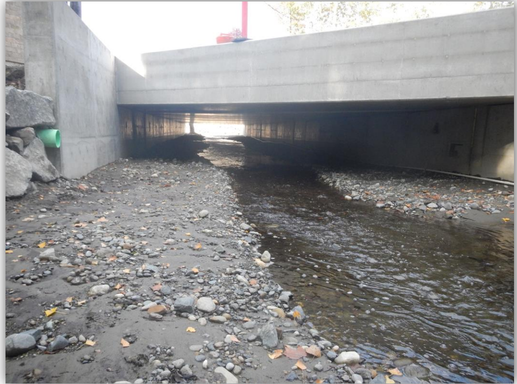
New 20 ft wide structure
