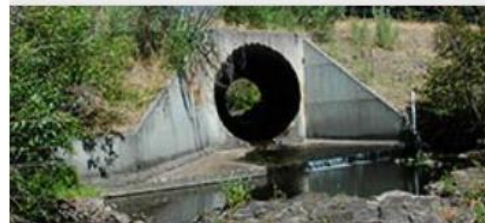
US 97 culvert that blocked fish passage at Butler Creek, a tributary to the Little Klidkitat River near Goldendale.
