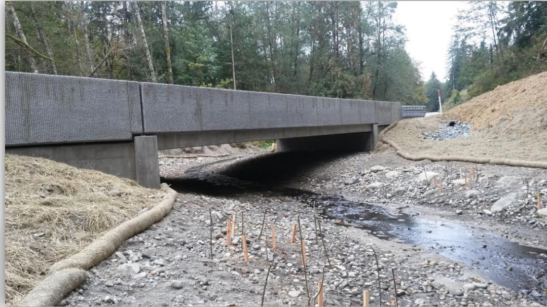
45 ft wide bridge
