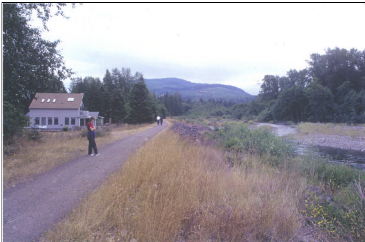
Figure 43. Right bank levee on Dungeness River, about 360 m (1200 ft) upstream of Hwy 101 (Photograph by Kondolf 2001).
