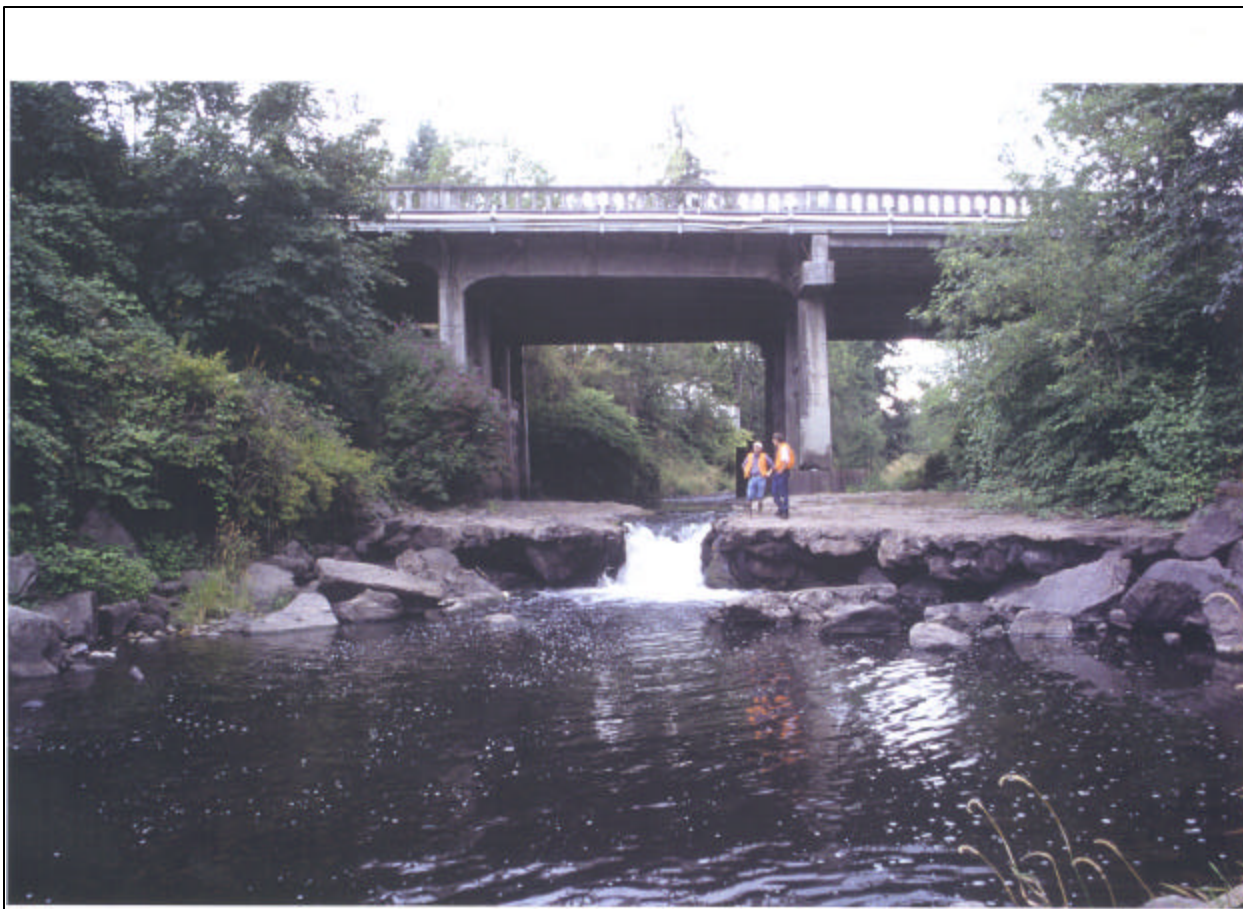
Figure 33. Headcut caused by regressive erosion upstream from captured gravel pit on Salmon Creek, near Vancouver, Washington (Photograph by Kondolf 2001).
