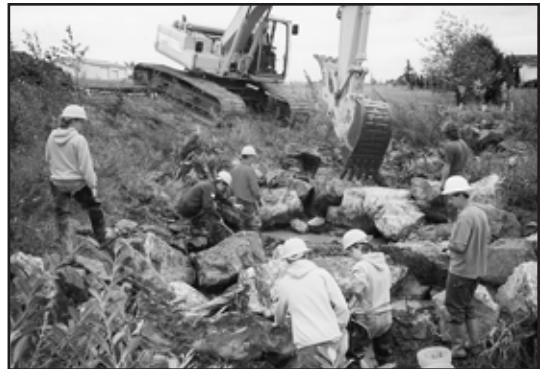
Photo: NSEA crew working on instream project.
