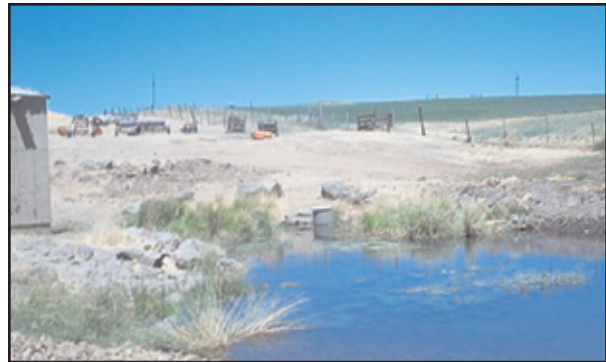
Blockhouse Springs 7/16/03 Post-Construction
