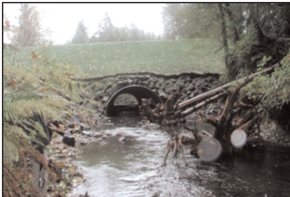
Unnamed Creek project after construction.
