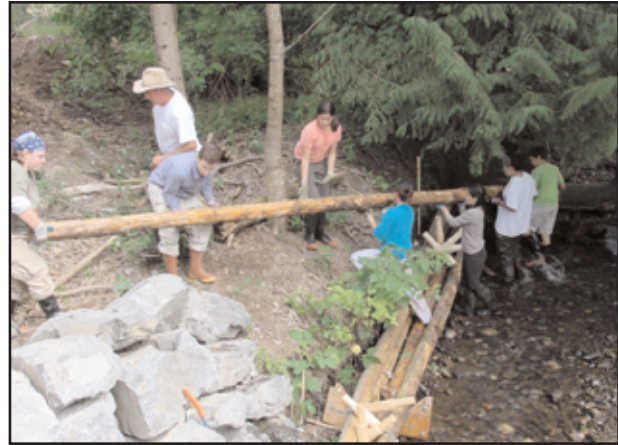
Volunteer installing ELWD structures in North Fork Newaukum Creek.
