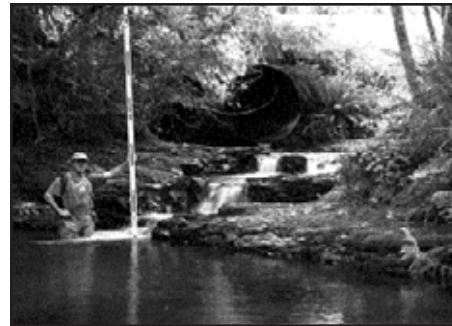
Oxbow Creek blocking culverts
