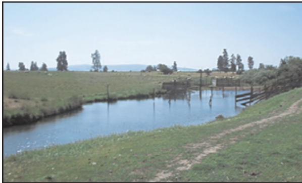
East on Blockhouse Creek-Enderby Project PRE-CONSTRUCTION 6/04/03
