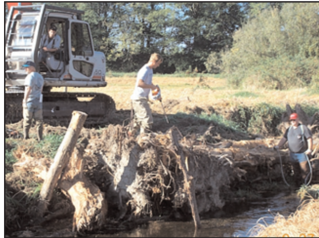
SFEG's restoration crew installing large woody debris at the East Fork Nookachamps project.
