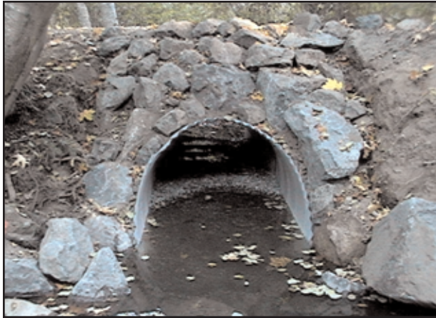
Completed Beachcrest Culvert looking upstream.
