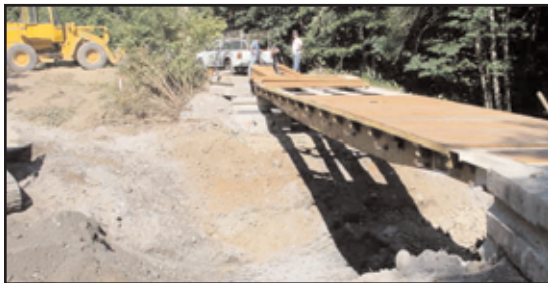
Bridge installation at the Valley Creek project site in summer 2002
