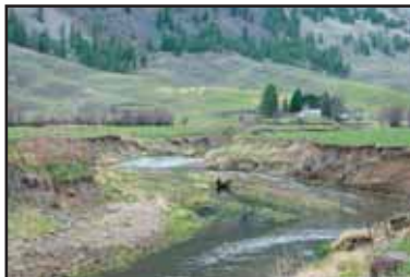
State of erosion along Sinlahekin Creek project area
