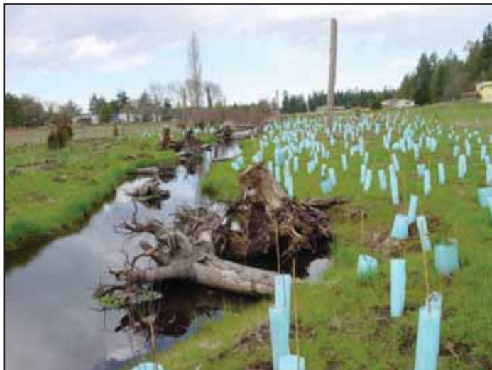
New restoration work completed along the east fork of Chimacum Creek.
