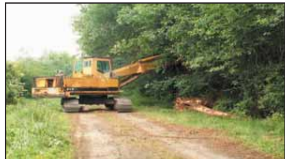
Equipment Placing Logs into Salmon Creek
