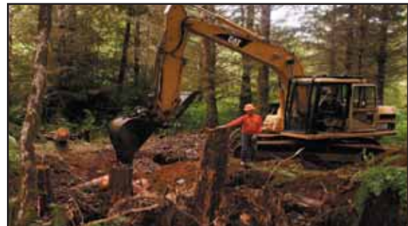
Placing Logs into position: Salmon Creek
