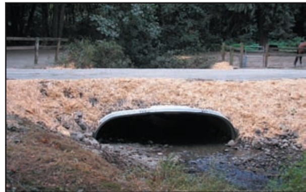
McKenna culvert post-construction.
