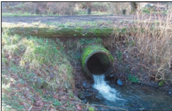
McKenna culvert barrier.
