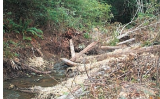
Lost Creek historic channel reconnected/restored
