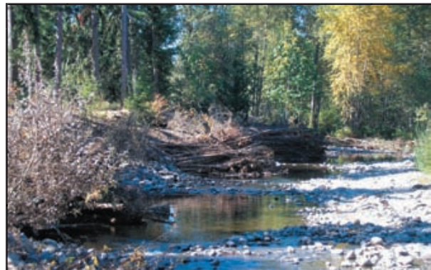
Mashel River ELJ #2, post-construction.
