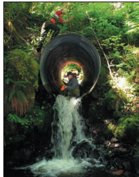
Two Earthwatch Institute volunteers measure a culvert that is a barrier to fish passage as part of a survey to assess salmon habitat above man-made barriers to fish passage.
