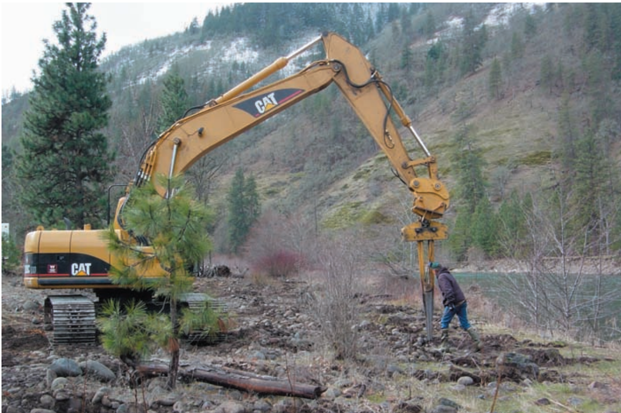
Planting along the Klickitat River using the hydraulic stinger, 2006.
