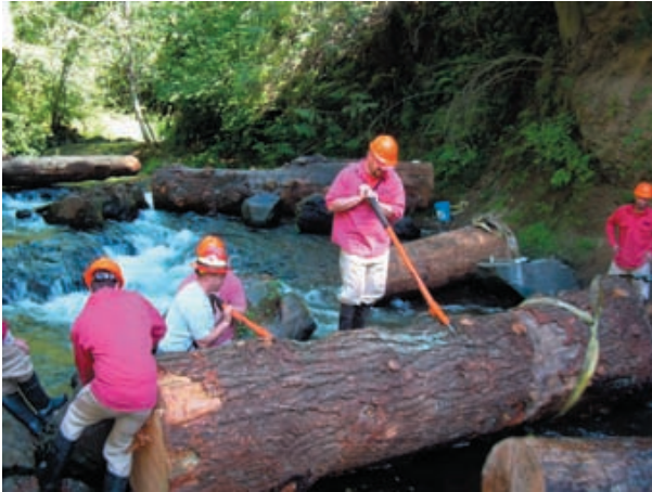
Crew positioning logs in Gobar Creek
