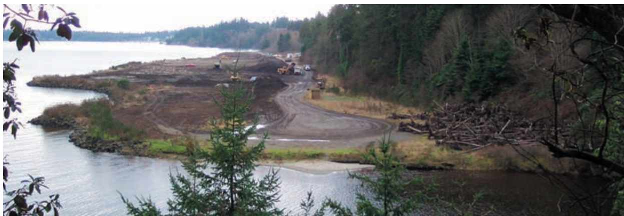
January 2006 — Chimacum Beach beginning excavation of fill.
