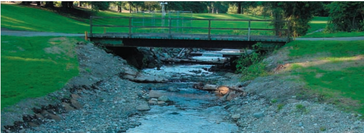
“Finished Instream Project on Kelsey Creek – Hole #6 at Glendale Country Club”
