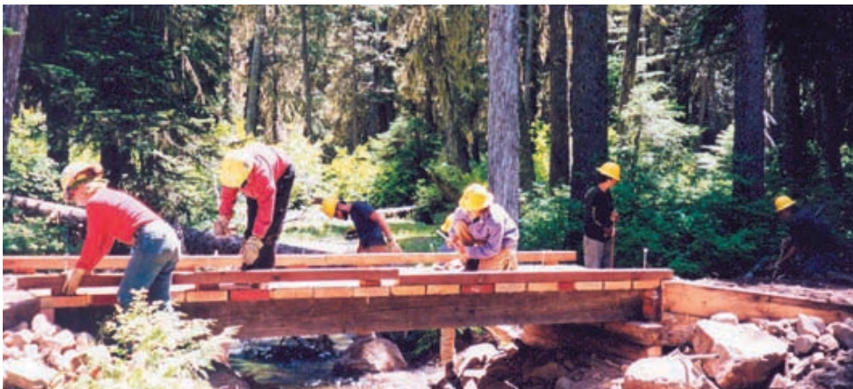
July 2005 – The Student Conservation Association Volunteer Crew replaces the culvert with a bridge using materials donated from the UCRFEG
