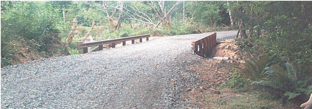
After New Bridge
