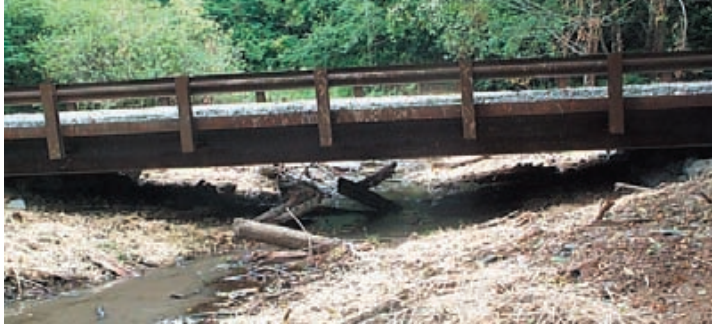
New Bridge/Channel on Lost Creek
