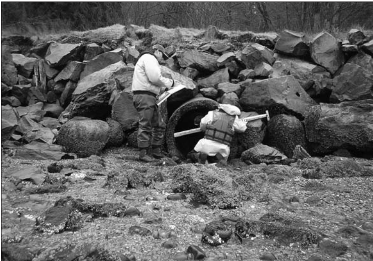
Nearshore Culvert Barrier Assessment.
