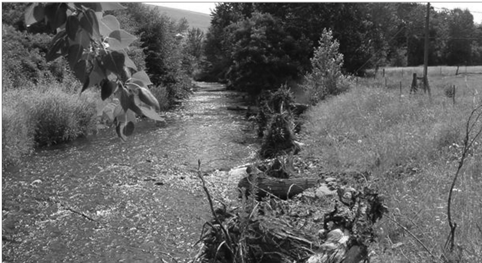
A rootwad revetment on the North Fork Touchet River has provided pools and habitat diversity previously lacking in this reach.
