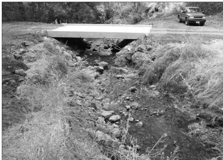
After – Culvert replaced by bridge to eliminate passage barrier.
