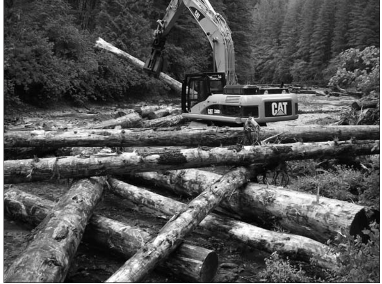
Placing logjam in upper Washougal River.
