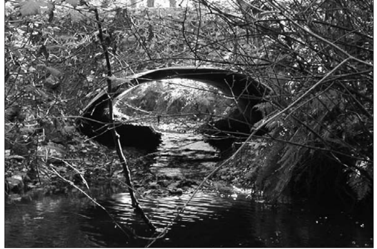
Freeman Dakota Creek culvert after.
