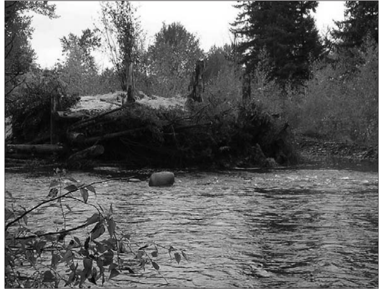
Engineered Log Jams on the Mashel River.
