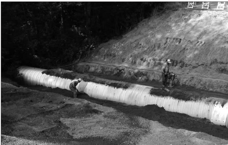
County Haynie Creek Culvert installation.
