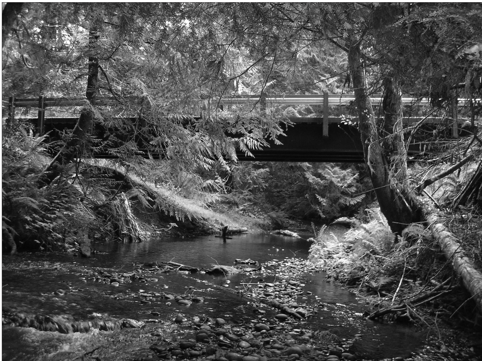
Huge Creek Bridge.
