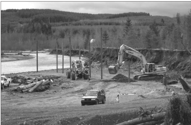
Bank stabilization on S. Fork Toutle River.
