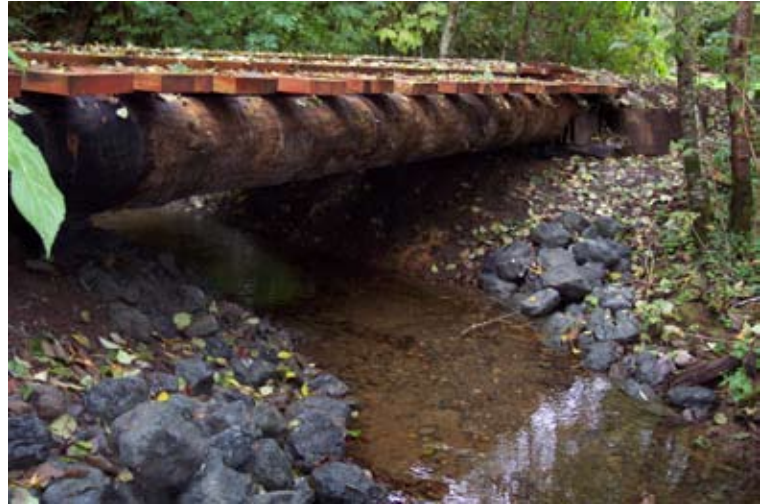
New log stringer bridge on Hammerquist creek.
