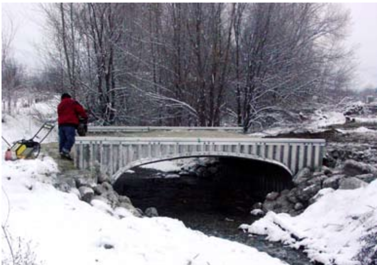
New bottomless aluminum box culvert on Antoine Creek.
