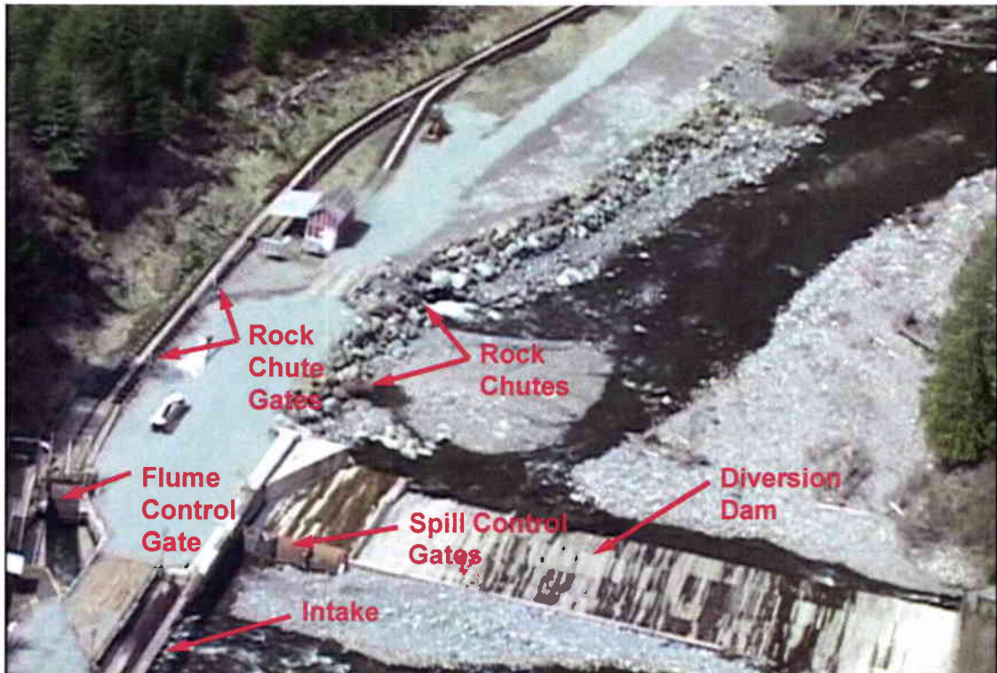
Figure 2. Features of the Electron diversion dam, intake, and beginning of flowline (Bates et al., 2008)
