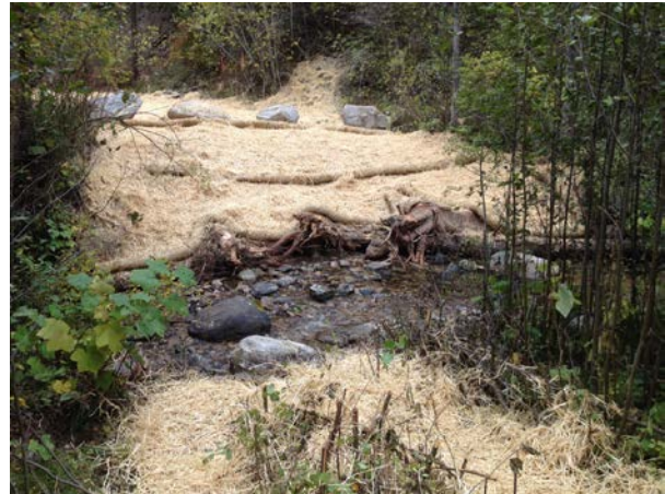
Completed bank stabilization on Trout Creek
