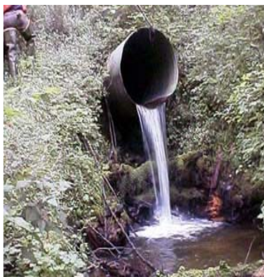
Figure 3-6. Drainage culvert projects are one type of activity contained in the HPMS database.
