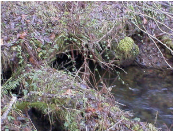
Photo 15. Site 980781, Shelton Creek (26.0640) tributary to Riffe Lake. This timber-made culvert is considered a partial barrier and may fail over time. Several timber-made culverts within this unit have failed, resulting in flow and passage obstructions.
