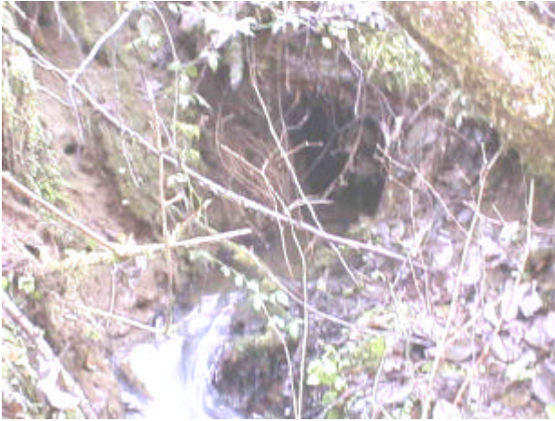
Photo 33. Site 980741. Unnamed tributary to Unnamed tributary to Riffe Lake. This timber-made culvert obstructs the flow and partially blocks fish passage.
