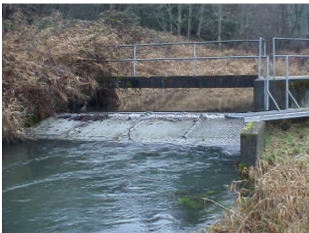
Photo 1. Site 981318, Blue Creek (26.0527) tributary to Cowlitz River. View of dam is obscured by the hatchery rack. The Fish ladder entrance is at the left bank. This site is a total barrier.
