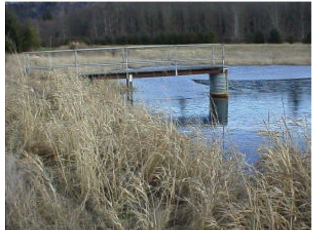
Photo 12. Site 980933, Unnamed tributary to Cowlitz River. Created for waterfowl enhancement, this dam site is a total fish passage barrier.
