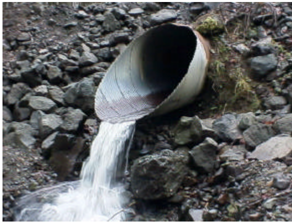
Photo 39. Site 980888, Riffe South, Unnamed tributary to Cowlitz River. This total barrier culvert is the only feature on this fish bearing stream and blocks access to approximately 736 linear meters of stream.
