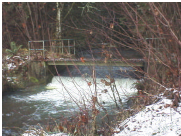
Photo 2. Site 980911, Blue Creek (26.0527) tributary to Cowlitz River. This dam is also equipped with a hatchery rack and is a total barrier to fish passage.
