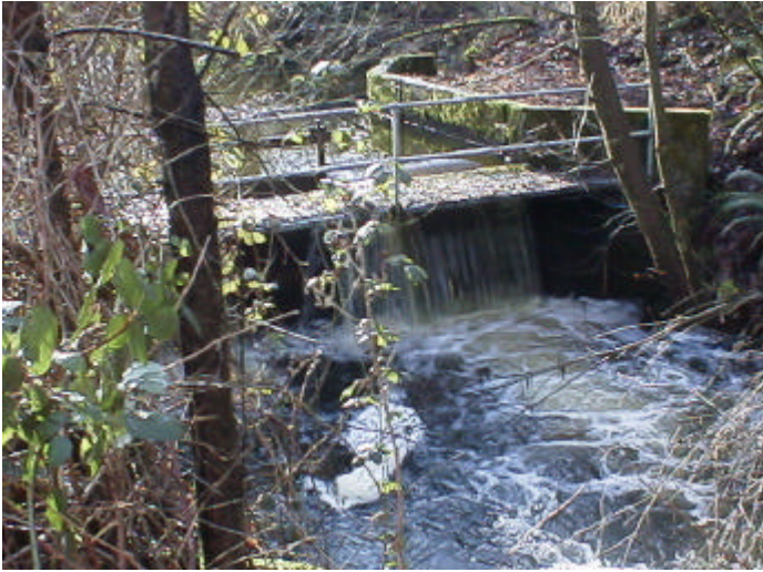
Figure 3. Site 01.0089 8.70, Lake Terrell Dam, is a total barrier to fish passage. Within the WLA, this is the only barrier on Terrell Creek. This dam blocks access to 8.3 km (5.2 miles) of stream habitat. The PI value for this barrier is 43.97.
