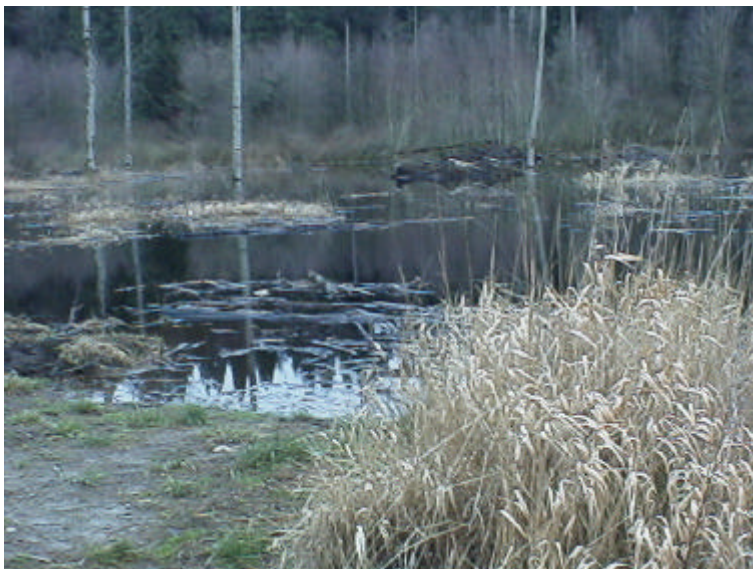
Figure 14. Site 981779 features an earth dam with a vertical standpipe to control water level. The photo shows a small portion of the earth dam at the bottom left and the pond created by the dam. The dam is a total barrier to fish passage. Fish use of the pond is likely limited to winter rearing due to high water temperature in summer. The pond has 3,364 square meters of potential rearing habitat. The PI value is 15.82.
