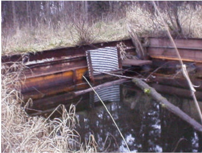
Figure 7. Site 981786 features an earthen dam with a headgate on a culvert. This total barrier to fish passage blocks access to 1.14 km (0.71 miles) of stream containing 12,396 square meters of rearing habitat. The PI value for this barrier is 21.91.
