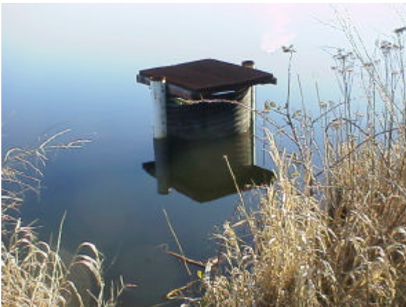
Figure 4. Site 981798 features an earthen dam with a vertical standpipe. This total barrier to fish passage blocks access to 2.0 km (1.23 miles) of stream containing 0 square meters of spawning habitat and 16,841 square meters of rearing habitat. The PI for this barrier is 23.65.
