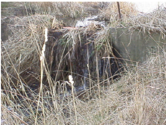
Figure 15. Site 981792. This concrete dam is just upstream of the confluence with Terrell Cr. Water spilling over the dam falls 0.90 meters onto a concrete apron. There is 4,084 square meters of potential rearing habitat upstream. This barrier has a PI value of 16.60.
