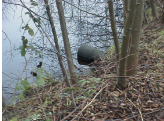
Figure 11. Site 981783. An earthen dam with a 0.21 meter overflow culvert creates a small isolated pond. The pond has 788 square meters of potential rearing habitat. The PI value for this total barrier is 3.12.
