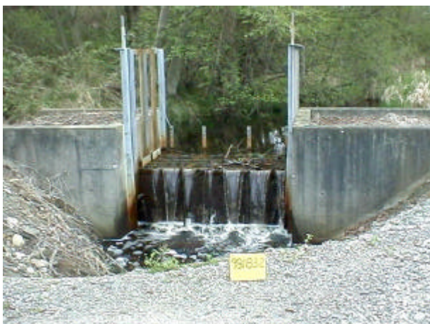
Figure 24. Immediately upstream of site 981830 is site 981832, which is a pollution control device consisting of hay bales inside of an expanded wire mesh cage. This feature acts as a dam blocking access to 0.66 km of stream and pond habitat. There is no spawning habitat upstream but there is 3,370 square meters of rearing habitat in beaver ponds and wetlands. The PI for this barrier is 15.82. This site is on BP land.
