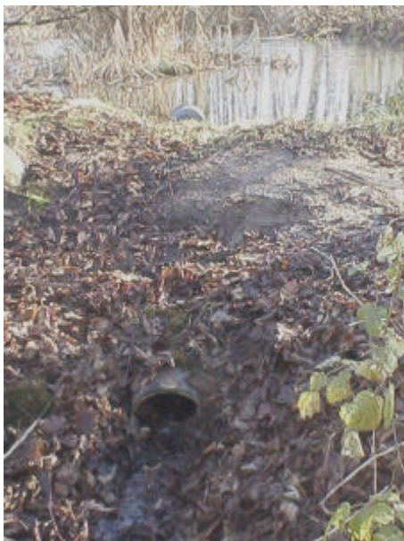
Figure 12. Site 981787. An earthen dam with a small (0.21m) overflow culvert creates a small isolated pond. The pond has 1,126 square meters of potential rearing habitat. The PI value for this total barrier is 3.41.
