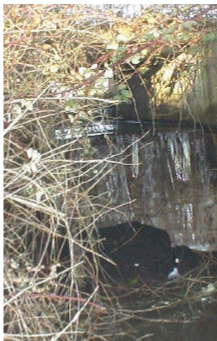
Figure 16. Site 981793. This site has an earthen dam with a concrete spillway and slots for stop boards. The spillway has a 1.54 meter outfall drop. There is 2,613 square meters of potential rearing habitat upstream. The PI value is 14.85.
