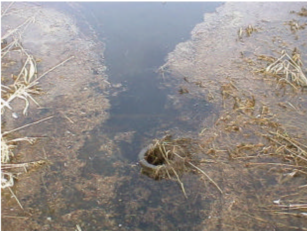
Figure 8. Site 981452, Shillapoo Lake to Lake River. Upstream view of dam spillway. Plywood is used to block inlet and a small standpipe is used to maintain the level of standing rainwater.
