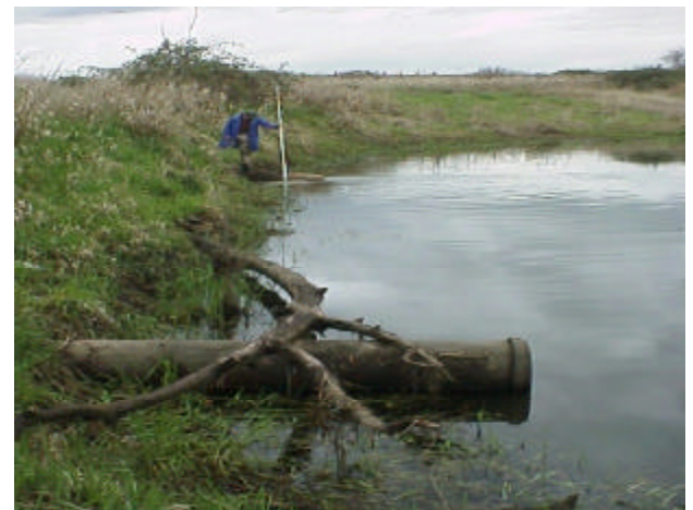
Figure 25. Site 981855 continued. Downstream view of smaller sequencer pipe near the right bank. No flow was observed during the outgoing tide. While both pipes become inundated during high tide, this smaller pipe is set at a higher elevation and becomes dry during low tides.
