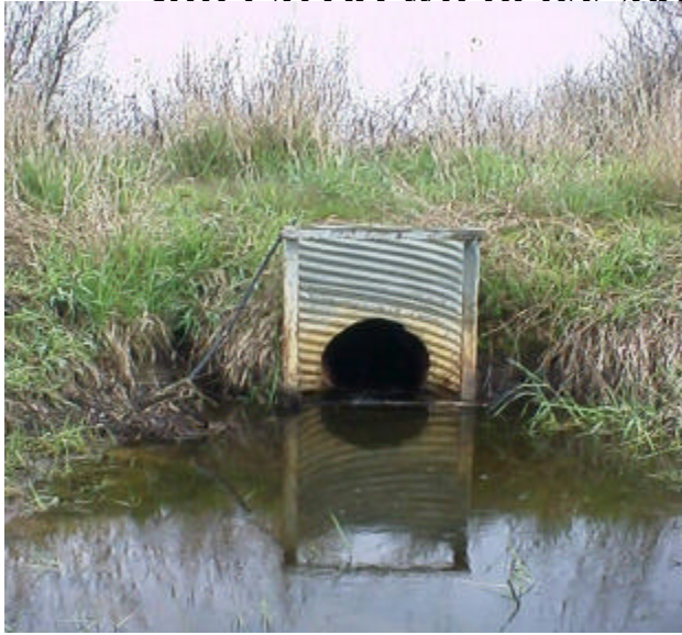
Figure 26. Site 981471, Mulligan Slough to Vancouver Lake. View of the inlet and water control structure. Placement of dam boards to impound water creates an outfall barrier. This site is the principal location of tidal influence.
