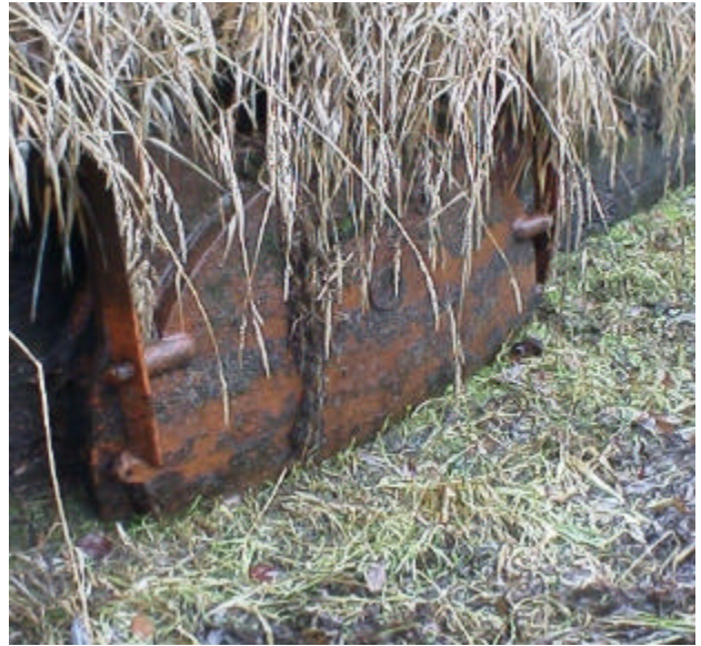
Figure 7. Site 981451 continued. Taken at low tide, this photo shows the sedimentation of the tide gate.
