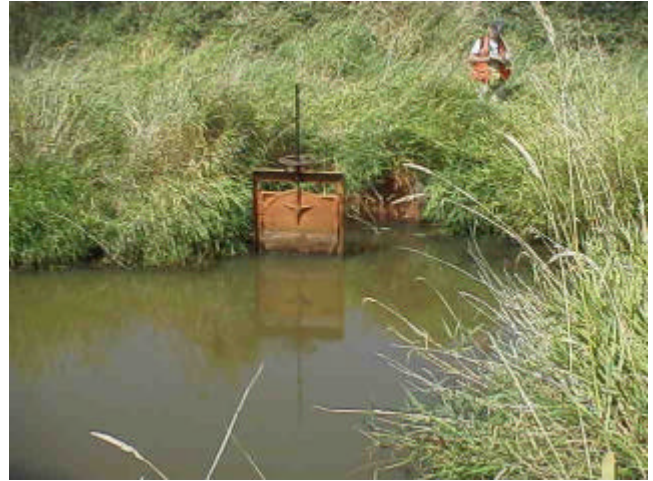
Figure 15. Site 981876, Unnamed to Deepwater Slough. This feature could be shut and potentially strand fish upstream. The artificial drainage upstream is a borrow ditch that follows the perimeter of the dike system. Site 981923, not shown, is upstream of this potential barrier.
