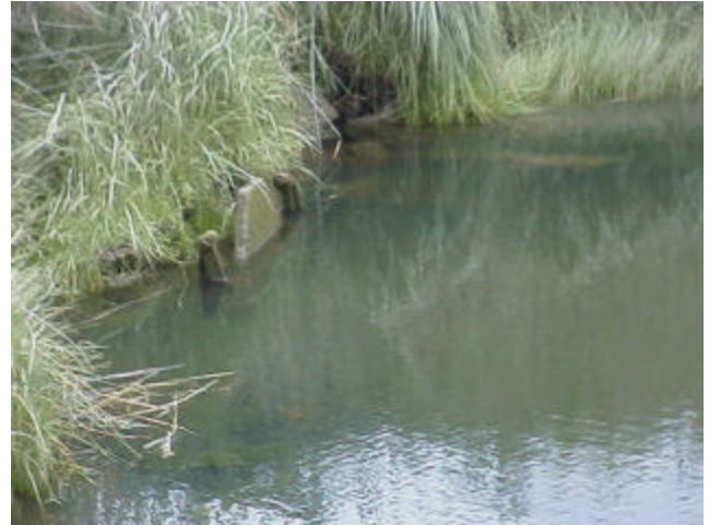
Figure 11. Site FI 9 continued. View of left bank tide gate.
