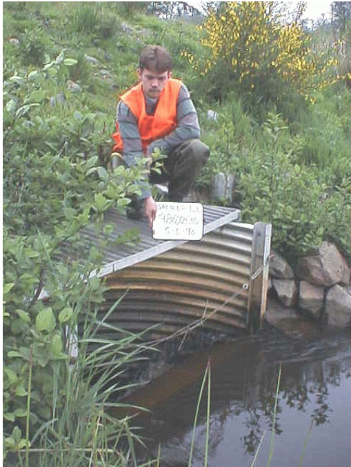
Photos 14 & 15. Wetland drainage. Installed through the dike, this large culvert is designed with a water level control structure on the upstream end and a tidegate on the downstream end, creating a barrier to potential summer rearing habitat.
