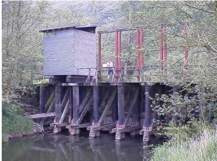
Photo 1. Pump house view from Wildlife Area side.
