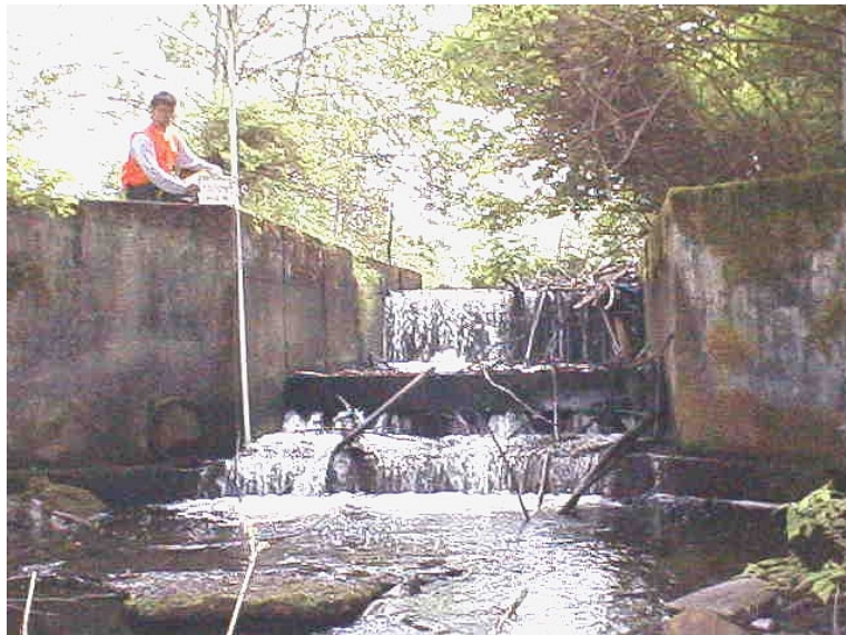
Photo 22. Bosworth Lake Creek (WRIA 07.0163). This feature was originally designed as a drum screen lake outlet structure. The screen has been removed and the structure is currently used as a lake level control device. Coho and other salmonids have been known to spawn immediately downstream. A pool and weir fishway is recommended.
