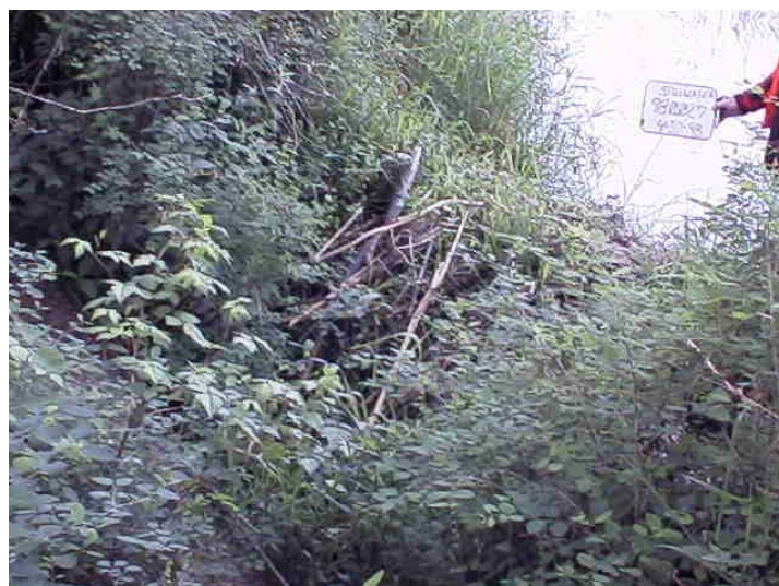
Photo 12. Unnamed tributary to Snoqualmie River. This small human-made dam was constructed to increase waterfowl habitat. At the same time it created a barrier for salmonids. Beavers have added to the size of the dam. The dam should be removed or a small fishway installed.
