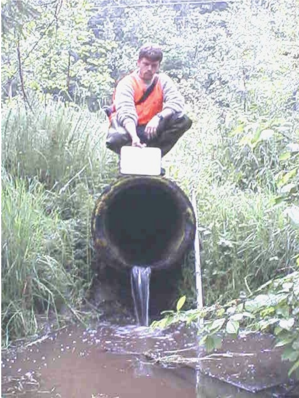
Photo 23. Dry Creek (WRIA 09.0089). There are several human-made barriers downstream of site 980051 and since the Forest Practices Appeals Board reversed DNR's determination that 09.0089 was a Type 3 water above 180 th Street and reclassified it as a Type 4, those additional barriers will probably not be addressed. If all human made barriers were repaired fish would probably move up the stream again.
