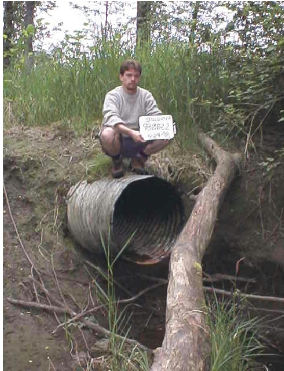
Photo 9. This large corrugated steel culvert is severely undersized for winter flows and has created a huge plunge pool, rendering the culvert a barrier to fish. The culvert should be replaced with a substantially larger one or completely removed to allow access to additional winter rearing.
