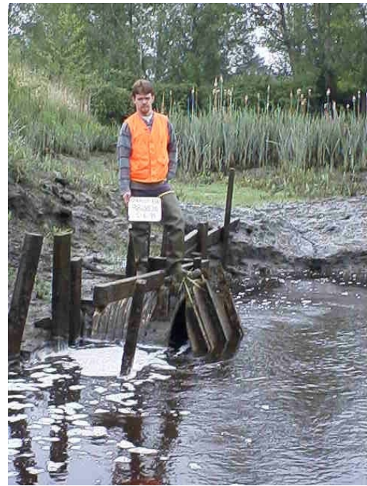
Photos 14 & 15. Wetland drainage. Installed through the dike, this large culvert is designed with a water level control structure on the upstream end and a tidegate on the downstream end, creating a barrier to potential summer rearing habitat.
