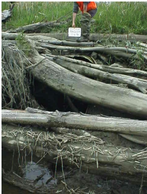
Photos 19 & 20. Identical design as Site 980038, the tidal side of the culvert / fishway is heavily influenced with tidal debris and the upstream end is designed for water level control, creating a barrier at various tide levels.
