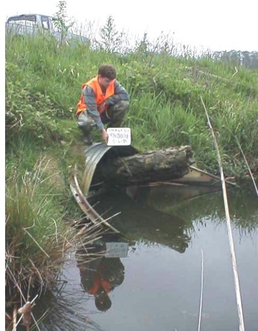
Photos 17 & 18. The photo on the left illustrates a flow control device installed on the tidal side and the photo on the right illustrates the large debris contributing to the barrier. This structure was designed as a flow control structure / fishway, but is still a partial barrier during tidal exchange and low tide.
