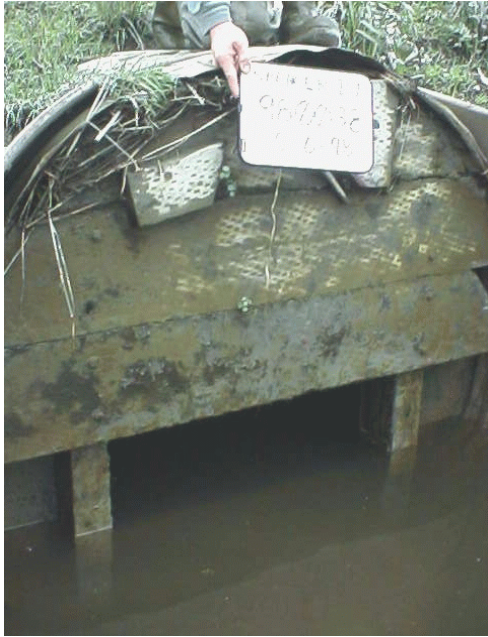
Photos 17 & 18. The photo on the left illustrates a flow control device installed on the tidal side and the photo on the right illustrates the large debris contributing to the barrier. This structure was designed as a flow control structure / fishway, but is still a partial barrier during tidal exchange and low tide.
