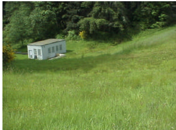
Figure 8. Site 981737. Building at base of Butterworth dam. Water flows from Butterworth reservoir down to Eden Creek reservoir.
