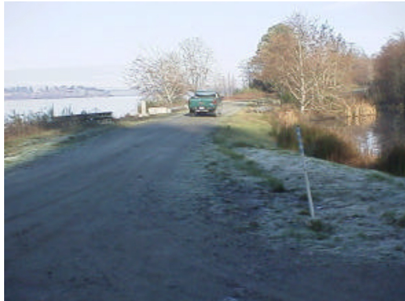
Figure 14. Site 981753. Coastal Road/Floyd Cove Dam. Reservoir on right, Pitt Passage on left. Overflow standpipe and culvert spill water into Sound.
