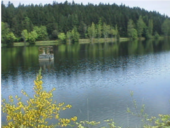
Figure 9. Site 981737. Offshore intake for Butterworth Reservoir which pipes water down to Eden Creek Reservoir.
