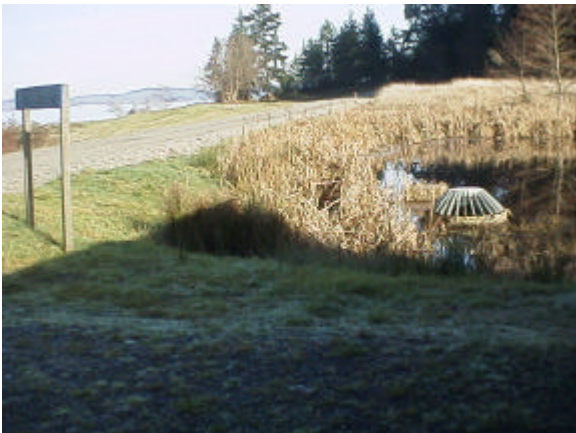
Figure 15. Site 981757. Bradley Reservoir on right with standpipe overflow. Puget Sound at upper left.
