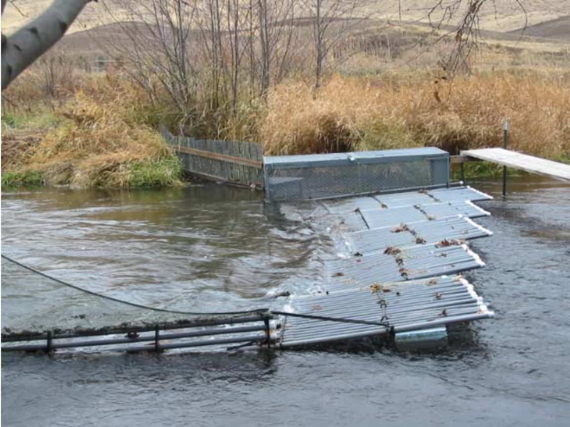
Plate 4. Digital photo of the redesigned steelhead weir and trap located at RM 10.3 on the Tucannon River. River is flowing from left to right in this photo, showing the floating picket panels and downstream migrant trap box.
