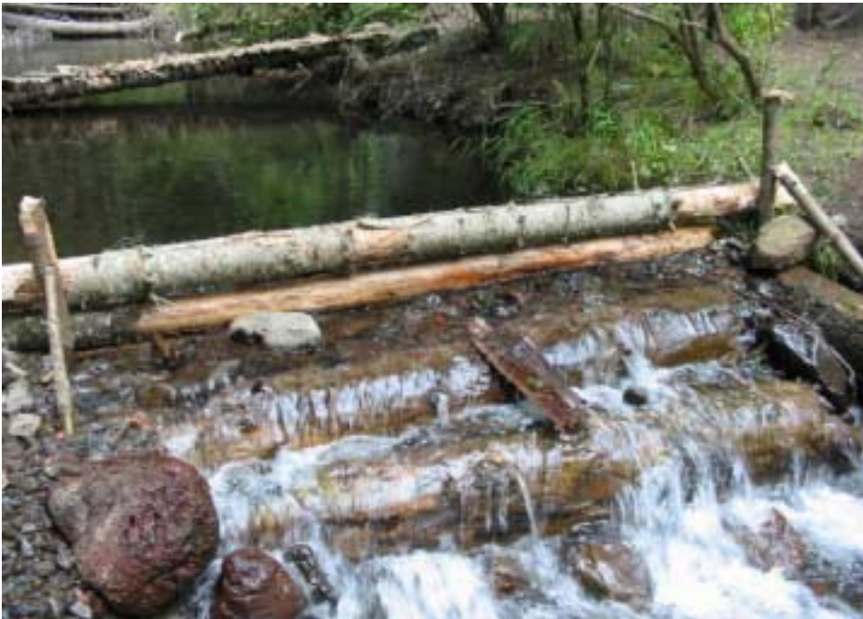
Plate 2. Digital photo of the dam built by campers on Panjab Creek, detailing the tight construction which impedes fish passage.
