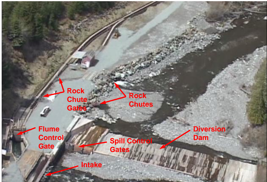
Figure 3. Features of the Diversion Dam and Flume Intake
