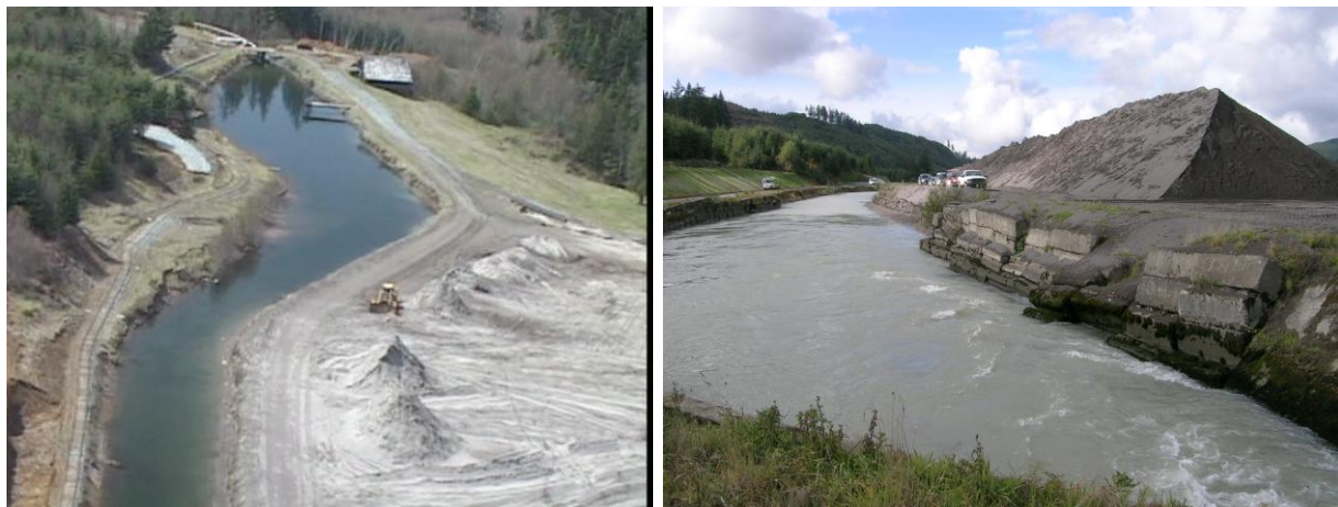
Figure 6. Settling Basin April 25, 2008 (left) and October 14, 2008 (right)
