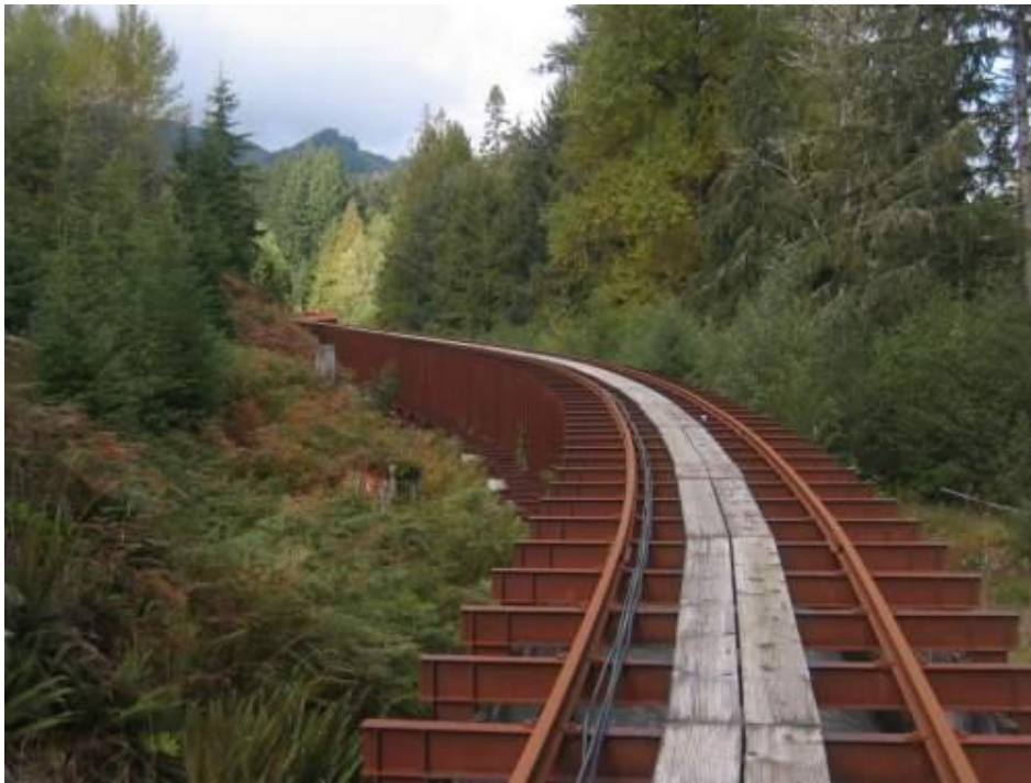
Figure 2. Electron Project Flowline Flume Section
