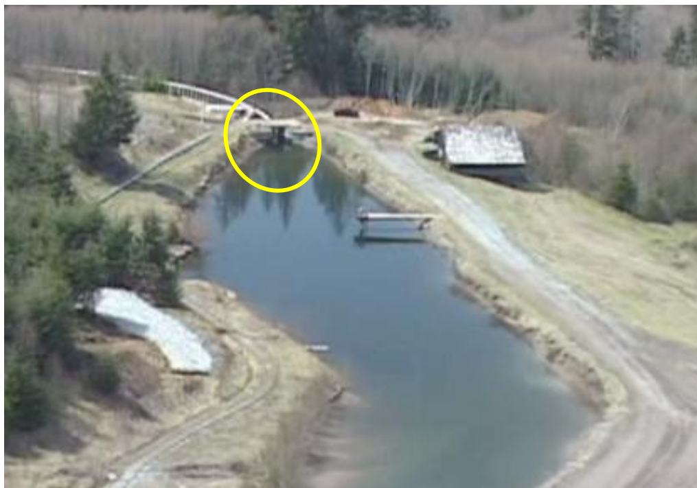
Figure 9. Downstream End Settling Basin
