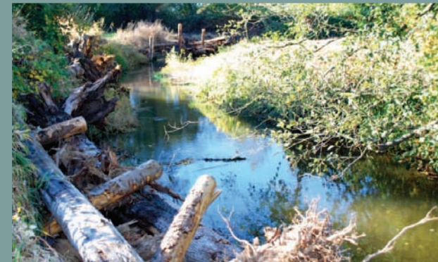
LARGE WOODY DEBRIS INSTALLED IN FISHTRAP CREEK
