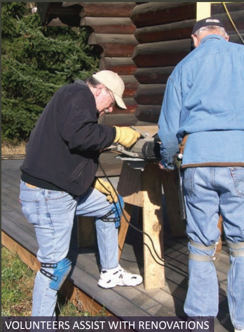
VOLUNTEERS ASSIST WITH RENOVATIONS
