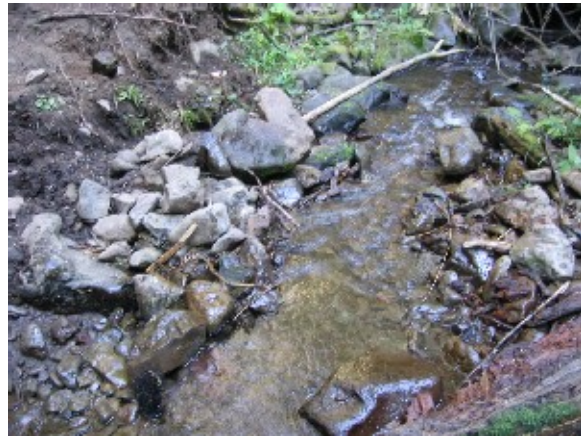
Photo 252. Upper man-made dam on Meadow Creek after it had been notched for fish passage, September 2007.
