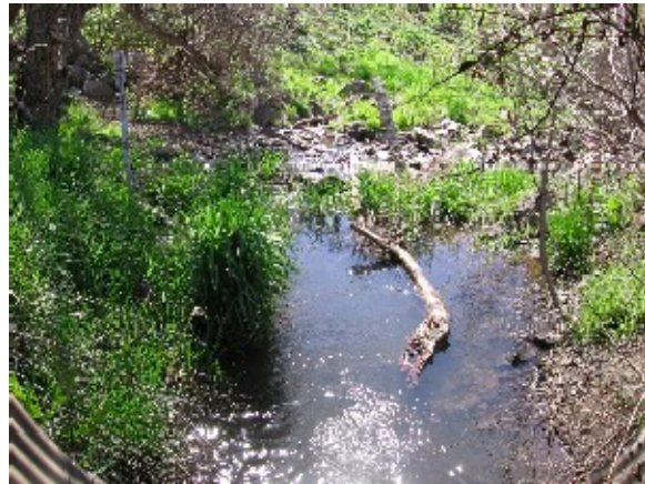
Photo 33. Shumaker Creek at first culvert above mouth looking out of the bottom of the culvert (SH-2), April 2007.
