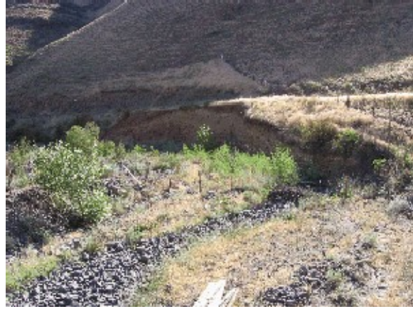
Photo 62. Couse Creek just below bridge on Couse Creek Rd. looking downstream, note dry channel, July 2006.
