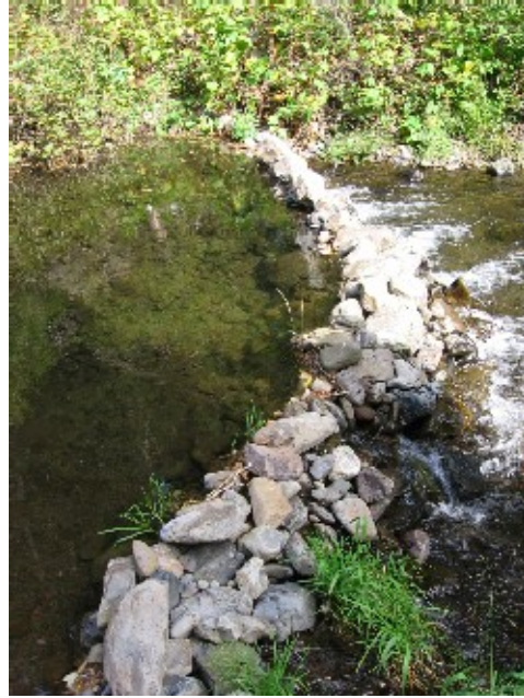
Photo 174. Side view of man-made rock dam seen in Photo 172, note grass growing on top of the dam, September 2007.
