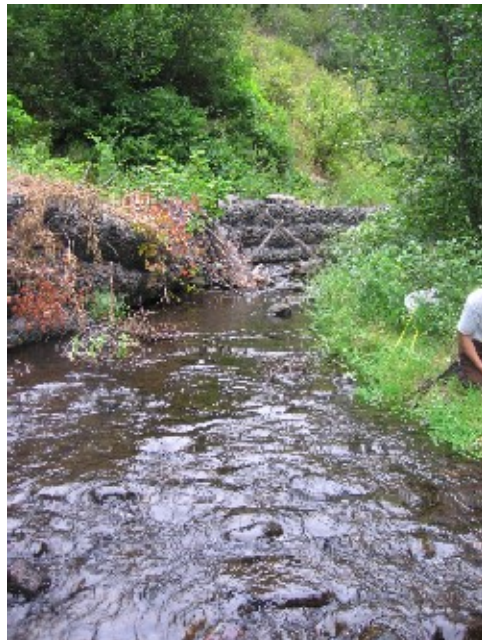
Photo 207. East Fork Butte Creek ~0.3 mile above confluence with West Fork Butte Creek looking upstream (EB-3) note gabion bank protection in background, August 2006.
