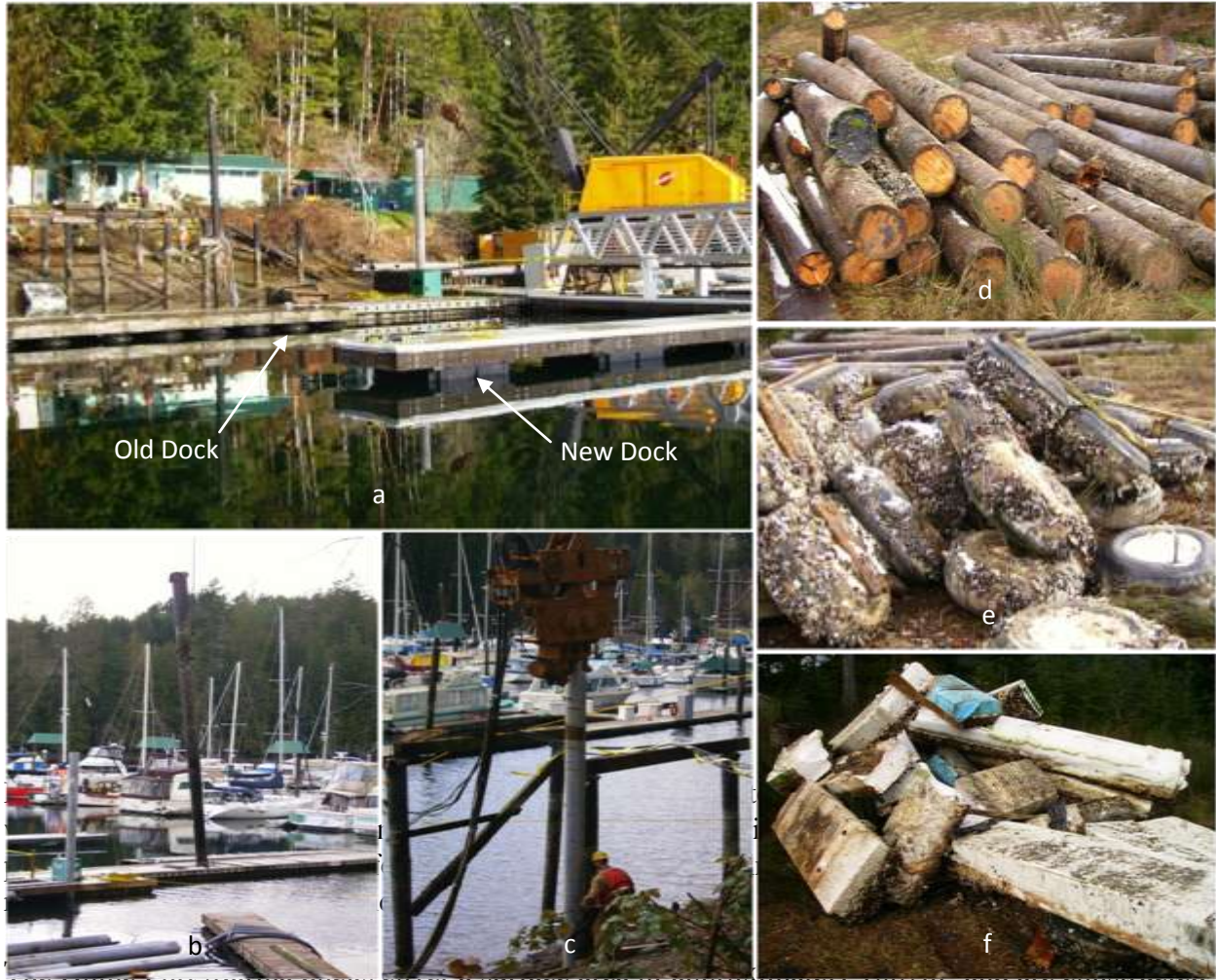
of foam-filled tires with wood deck surfaces held in place by 53 wood pilings. There is no covered moorage (Figure 18).
