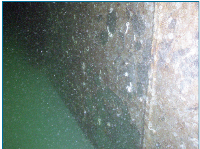
Figure 5: Concrete dock before and after pressure washing. Jesse Schultz, WDFW
