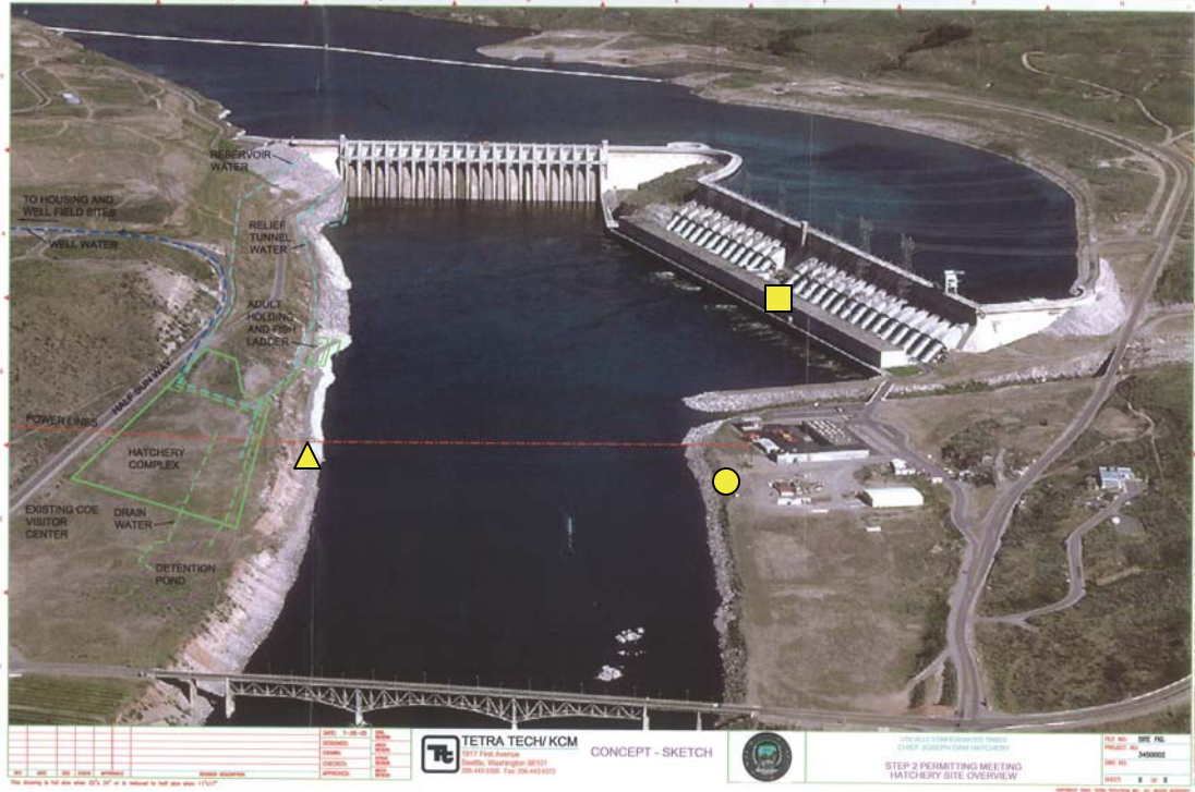
Figure 1. Photograph of the Chief Joseph Dam showing proposed hatchery site and ladder as well as location of radio telemetry fixed receiver Site 01 by a square, Site 02 by a circle, and Site 03 by a triangle. Photograph provided courtesy of Tetra Tech/ KCM.
