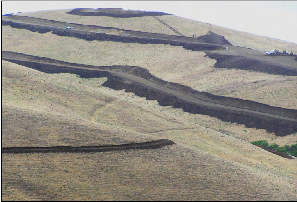
Figure 32. Access roads being prepared for wind turbines in Klickitat County.
