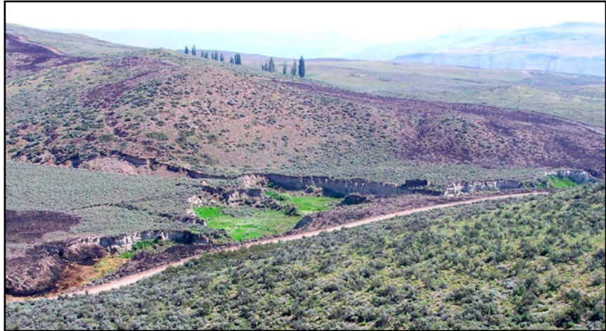
Figure 17. Down-cutting in Fye Draw near West Foster Creek in Douglas County.
