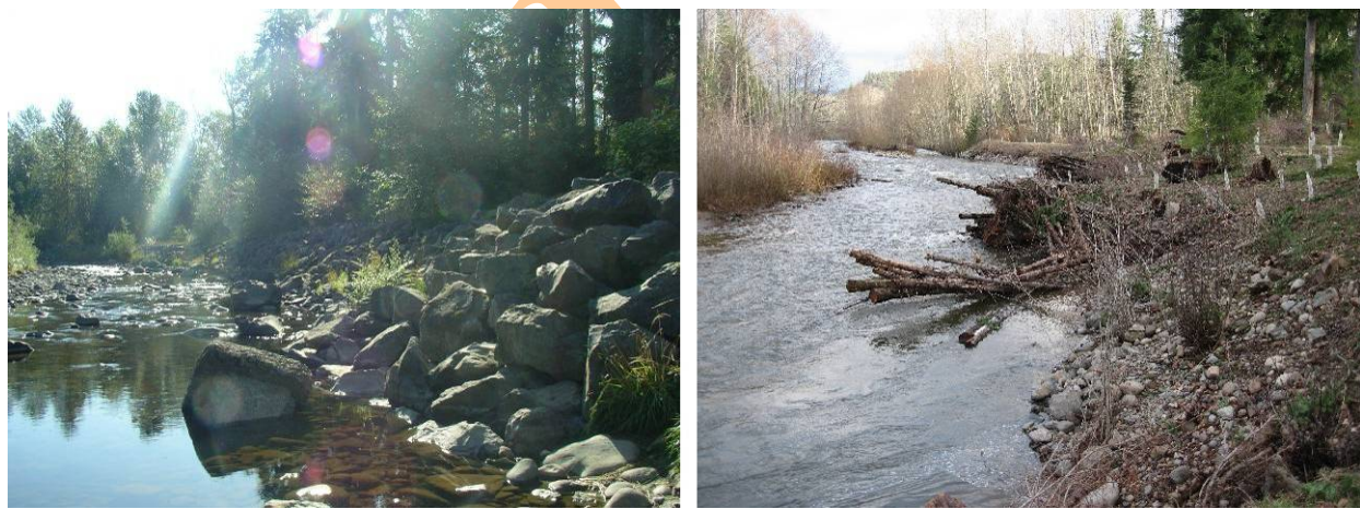
Figure 11-2. Example of bank protection before (left) and after (right) removal of the rock revetment and installation of engineered logjams in the Mashel River near Eatonville, Washington.
