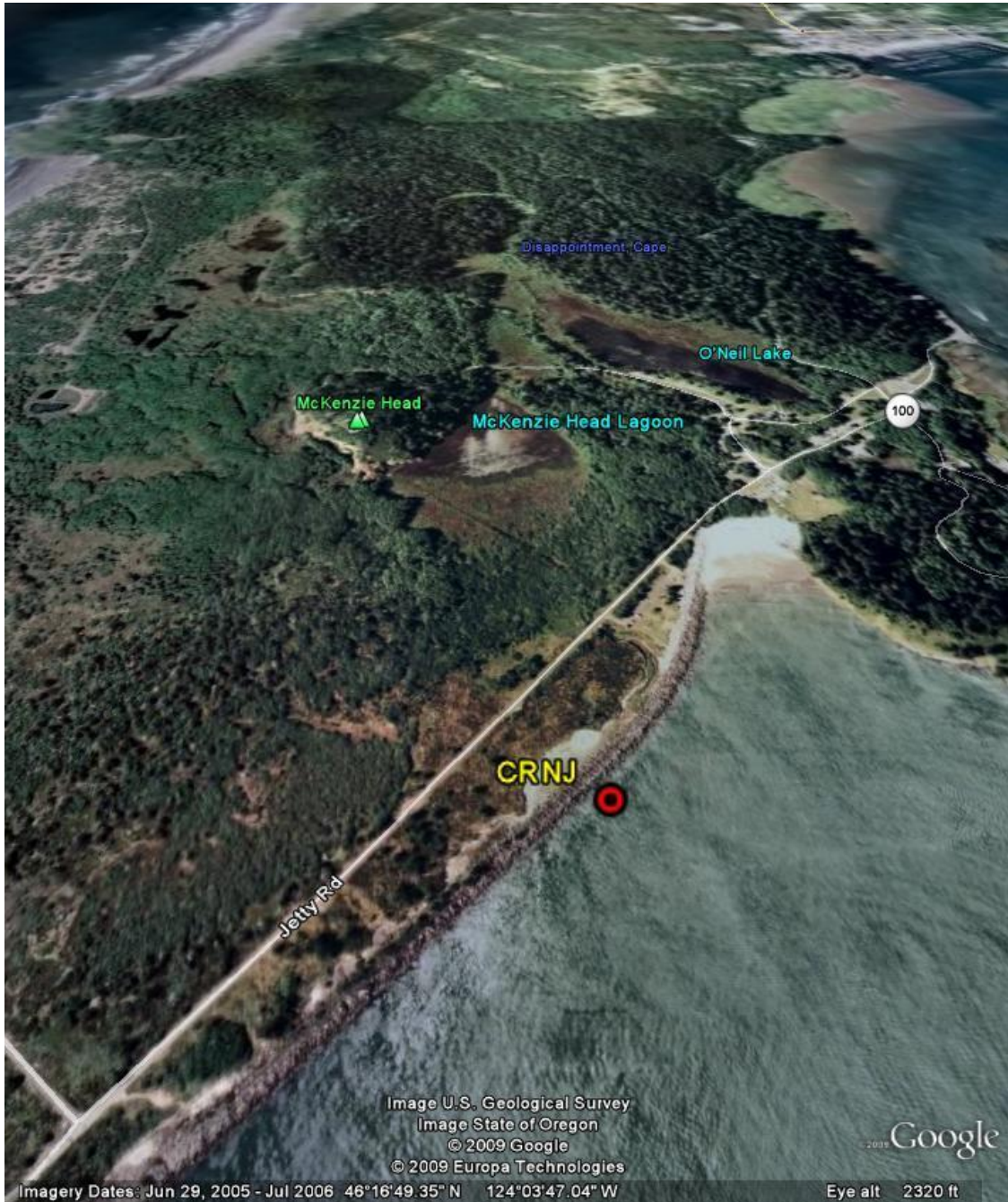
Aerial view of Columbia River - North Jetty (CRNJ) site.
