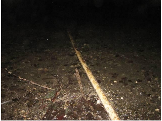
Stormwater outflow and PVC drain pipe running out of a buried location on upper beach and into the marine water near sampling location at SSBI site.
