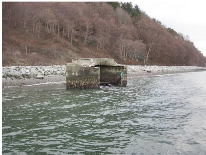
Concrete structure near PSHI site center.
