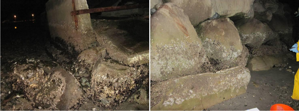
Concrete and natural rock construction of some retaining walls at sampling stations for CBTP site; creosote retaining walls not shown.
