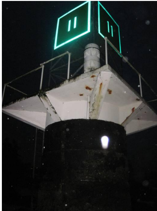
Navigation/channel marker (#11) at new Site Center of SIWP site.
