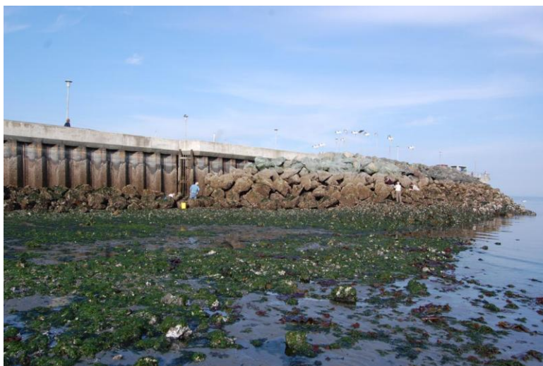
Breakwater at Puget Sound – Edmonds Marina (PSEM) site. Photo taken August, 2009.
