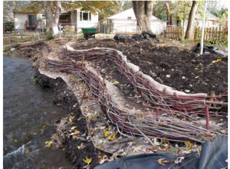
Willow Wall - One of our CURB projects
