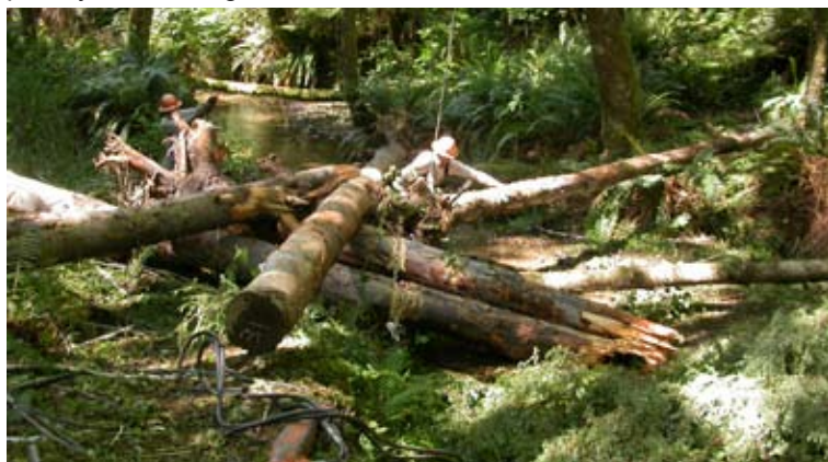
Large woody debris placement into South Stream
