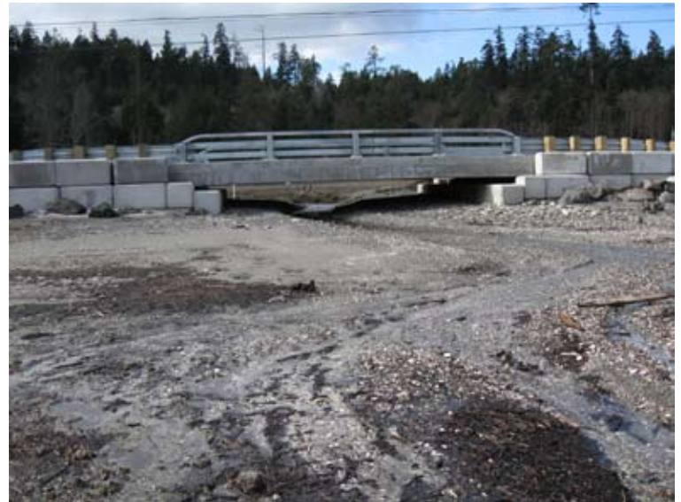
Pitship After: The restored Pitship Pocket Estuary with a 28-foot bridge that reconnects Sequim Bay with the estuary and restores access for out-migrating ESA-listed Hood Canal Summer Chum
