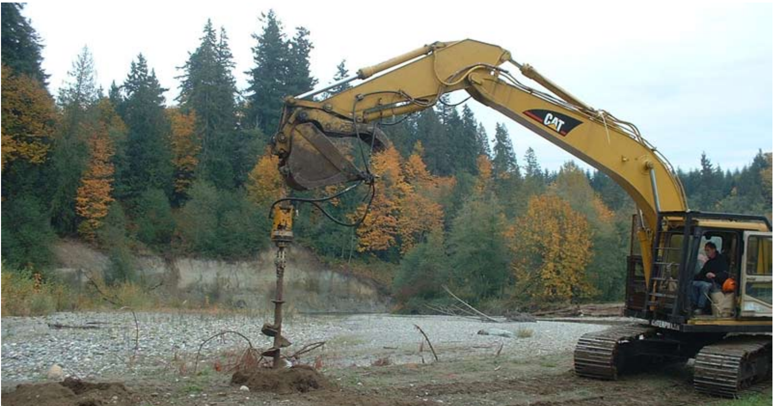
Heavy Equipment preparing to install flood fencing along the Pilchuck River
