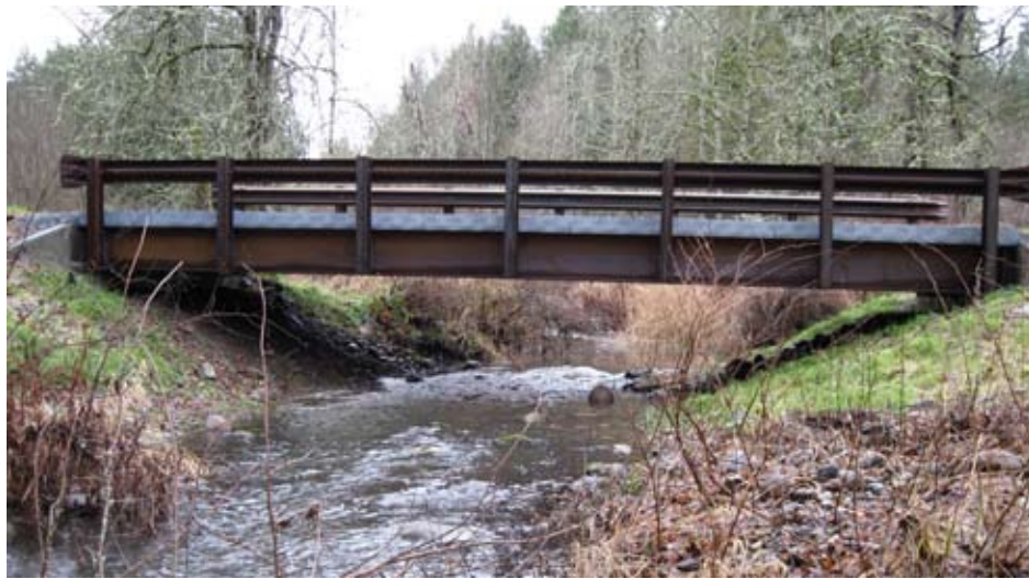
Thirty foot steel bridge on Lackamas Creek
