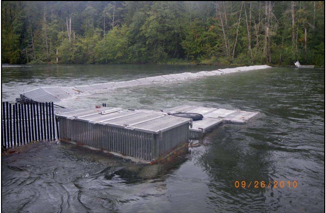
Figure 6. The floating weir operating at 2,190 cubic feet per second in the Elwha River on September 26, 2010 (USGS gage #12045500).
