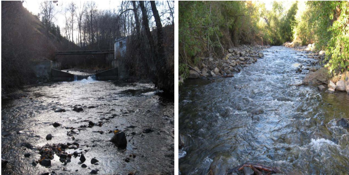
Figure 6. Diversion weir (left) replaced by roughened channel / constructed riffle (right). North Fork Ahtanum Creek, WA.
