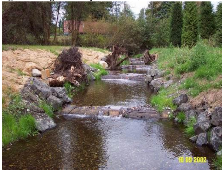
Figure 2. Log weirs. Hylebos Creek, WA.
