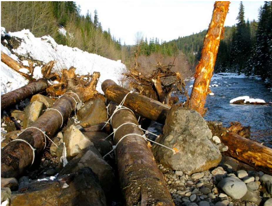
Figure 15 Logs cabled to boulder ballast (Klickitat River, WA, Inter-Fluve, Inc.).
