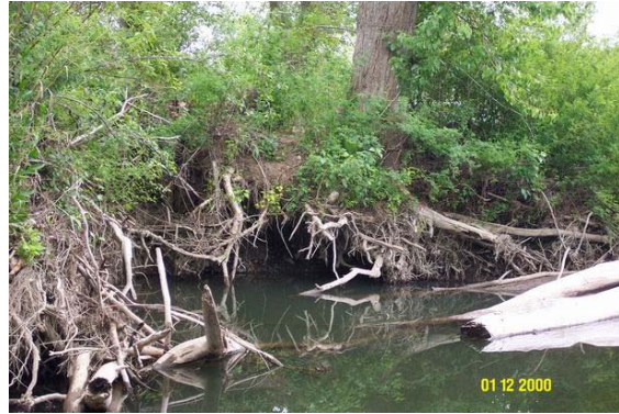
(b) Local scour creates small-scale complexity
