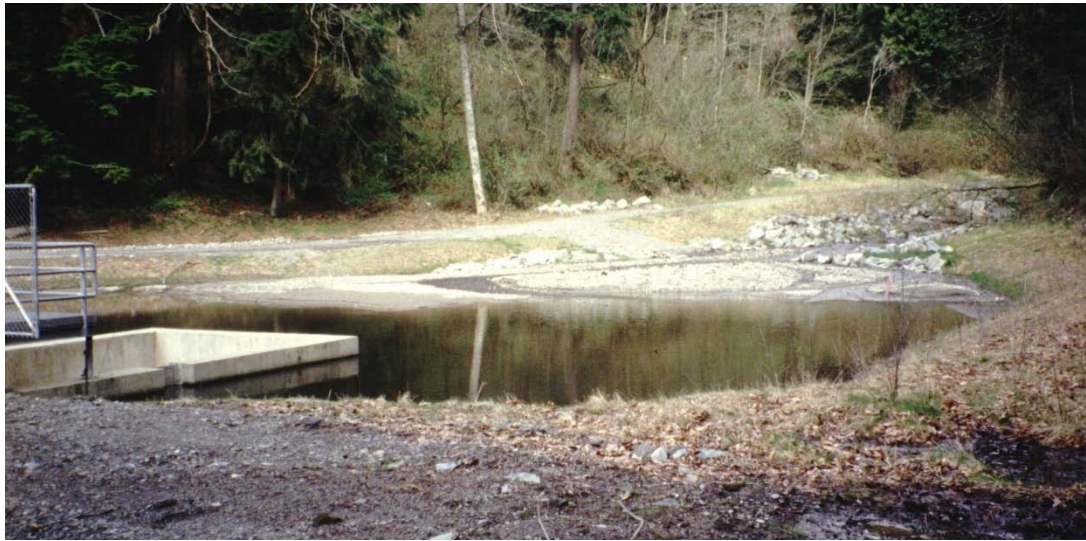
Instream Sediment Detention Basins Figure 6: Maplewood Creek sediment basin, King County. Looking upstream at sediment basin. High flow overflow structure in on right, inlet stream on right. Low flow outlet structure is a fishway off the picture on the left.
