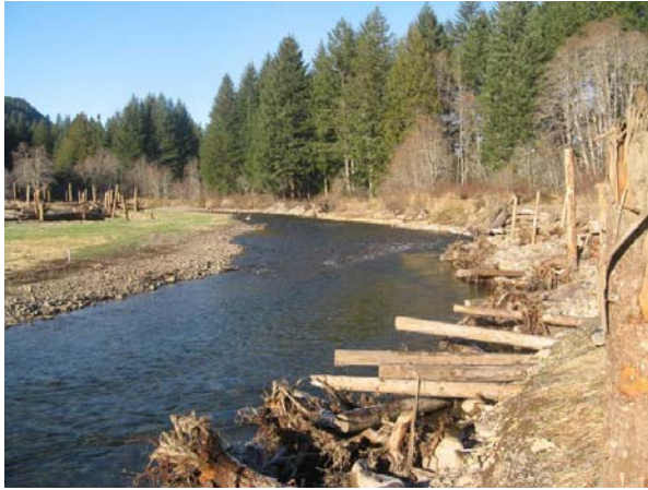
Figure 12. Reconstructed channel segments in the former reservoir of Hemlock Dam; Trout Creek, WA (Inter-Fluve, Inc.).
