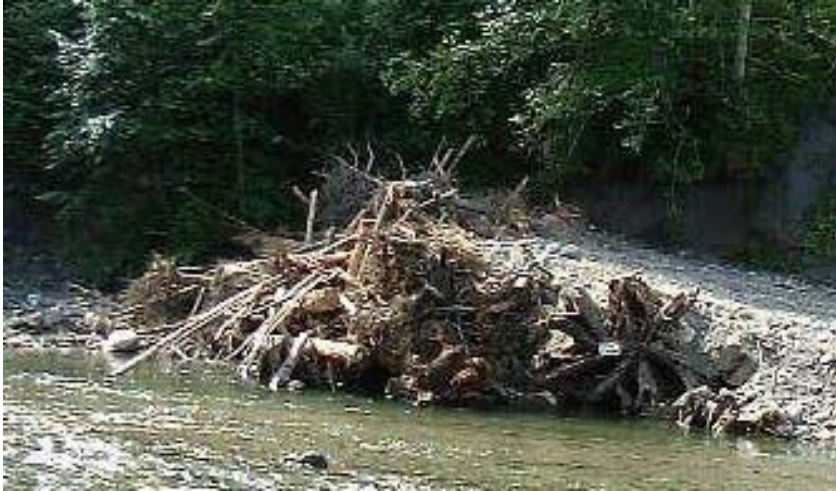
Figure 4. Log jam using gravel ballast (North Fork Stilliguamish River, Snohomish Co., WA).
