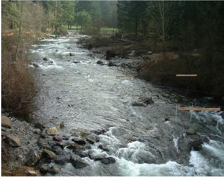
Figure 4. Porous boulder weir. Cedar River, WA.
