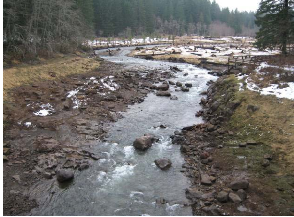
Figure 12. Reconstructed channel segments in the former reservoir of Hemlock Dam; Trout Creek, WA (Inter-Fluve, Inc.).
