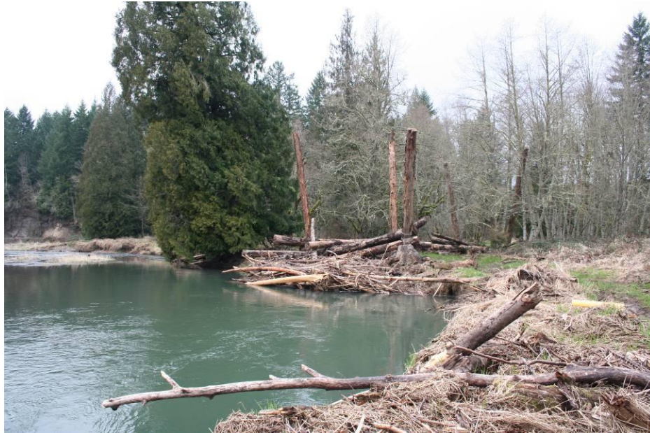
Figure 17. Collection of additional wood on a constructed meander bend log jam (Clear Creek, OR, Inter-Fluve, Inc.).
