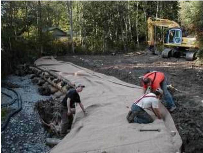
Figure 2. Spider Excavator placing rocks and logs in Whatcom Creek. Source: Inter-Fluve, Inc.
