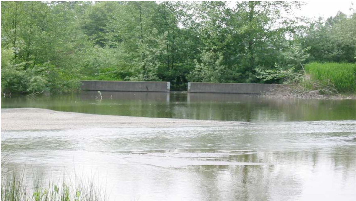
Instream Sediment Detention Basins Figure 2: Coal Creek sediment basin, Skagit County. Looking downstream from basin to slot-type outlet structure. Stream enters on left, deposition shoaling in middle left.
