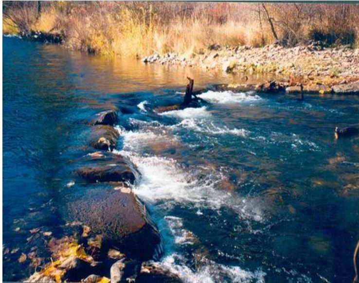
Figure 1. Rock weir. Cedar Creek, WA.
