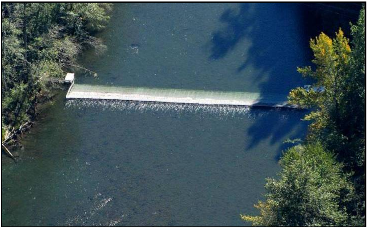
Figure 2. Floating weir in the Elwha River on the Olympic Peninsula in Washington State.
