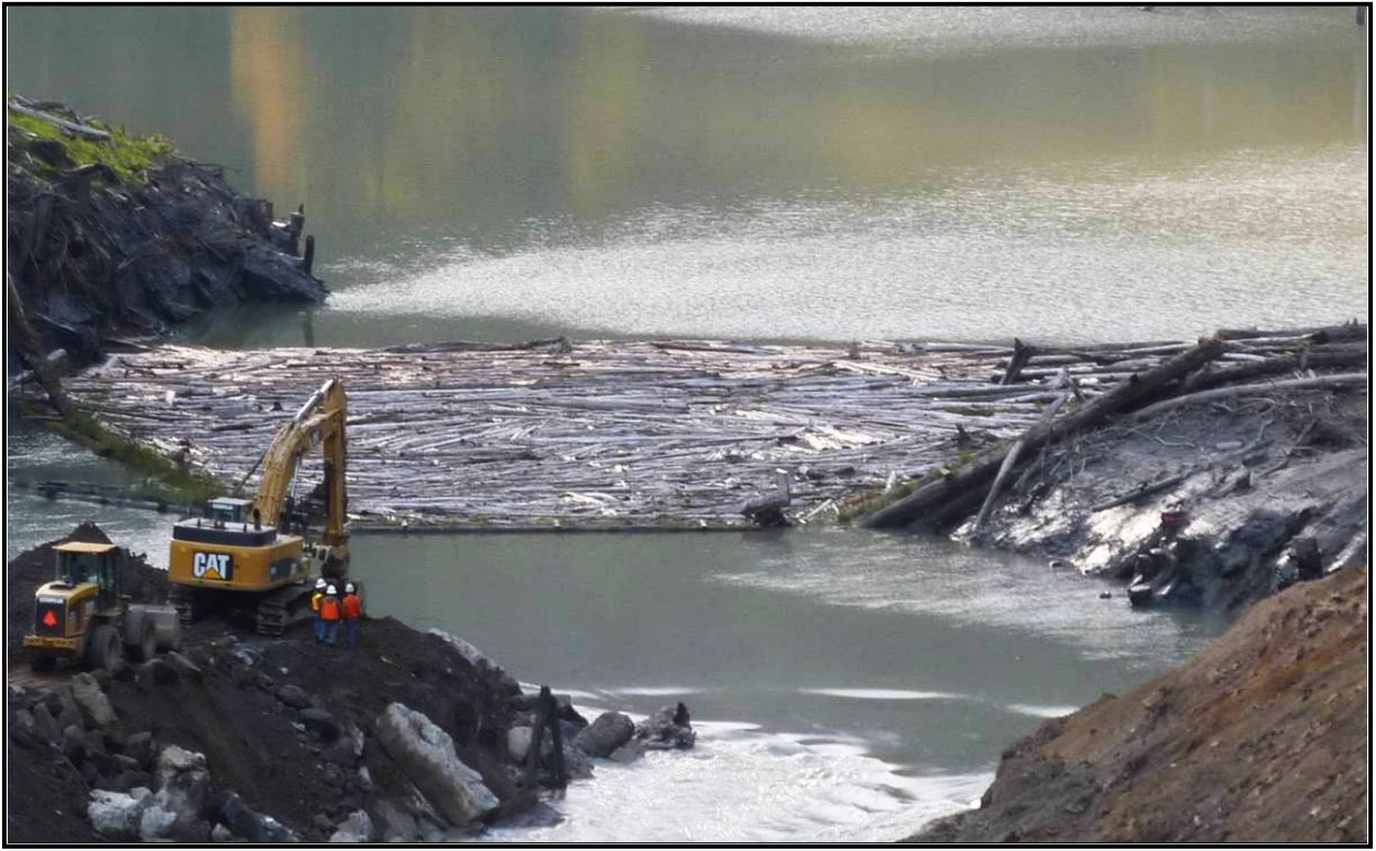
Figure 9. Hundreds of large logs at the Elwha Dam were released on October 21, 2011, which headed downstream into the lower Elwha River, in the direction of the weir (2 km downstream). The weir was removed one day prior to protect it from potential damage caused by the release.
