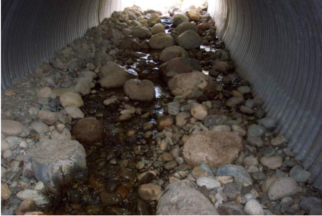
Figure 6.8: Roughened channel culvert. Shown at low flow. Bed material is rounded, but the bed should be countersunk deeper to be more robust.
