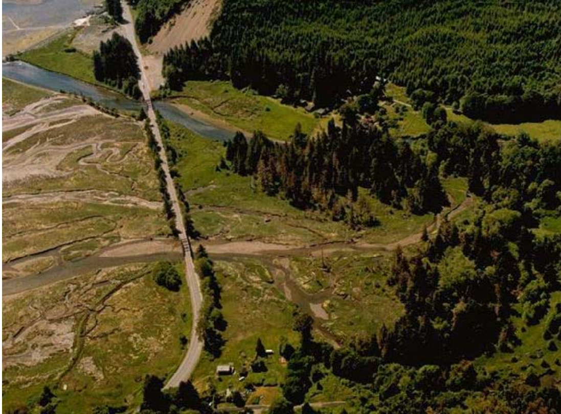
Figure D.1: US 101 crossing of the Hama Hama River delta (Washington Dept. of Ecology photo).
