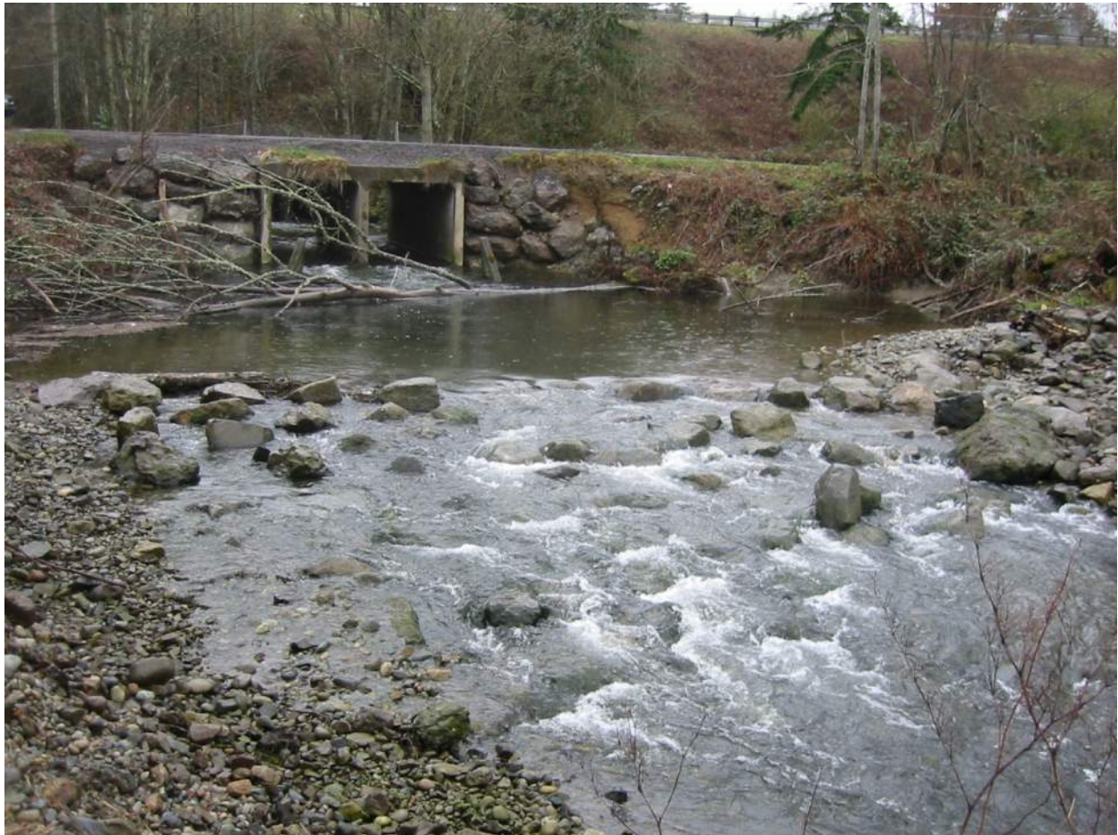
Figure 7.5: Constructed cascade used to backwater an existing culvert, Chico Ck.
