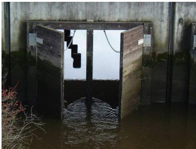
Figure 10.2: Above, hydraulically-controlled automatic tide gate, and (right) a float controlled automatic tide gate, both at Julia Butler Hansen Wildlife Refuge. Wooden barn door, side hinged, tide gate, below.
