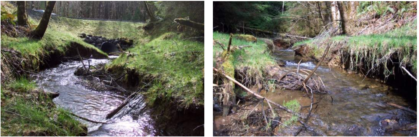
Figure 7.2: Regrade resulting from culvert replacement.
