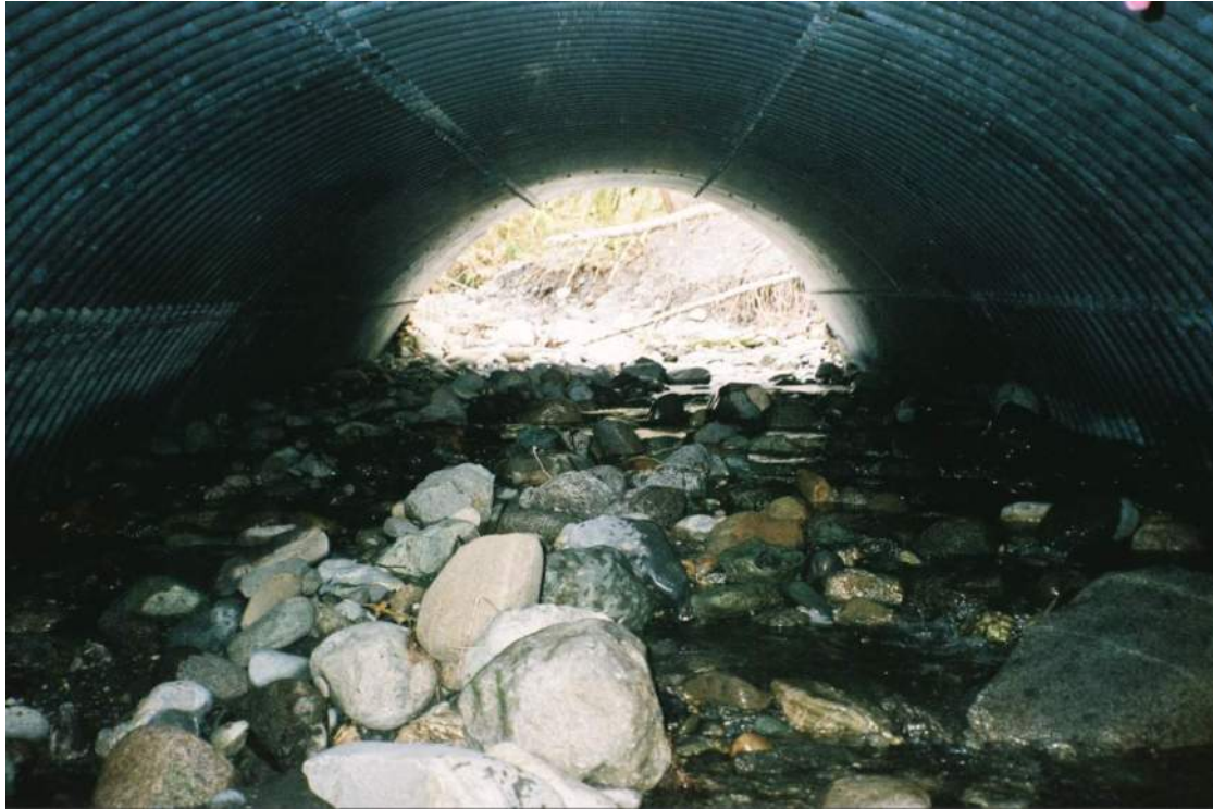
Figure 6.3: Roughened channel inside a culvert (photo Paul Tappel).
