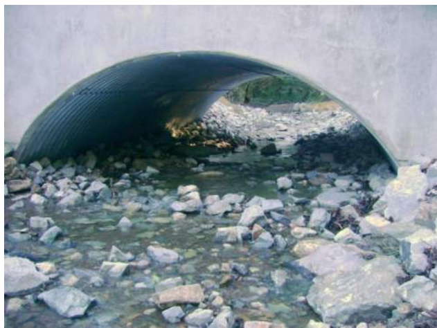
Figure 6.6: Roughened channel culvert in California, photo Michael Love and Associates. Bed is composed of angular material, which is the least preferred, and stream banks could have been reinforced with biotechnical methods rather than rock.
