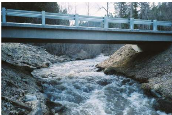
Figure 5: Roughened channel under bridge, Buck Ck, 2007 (photo, Paul Tappel).
